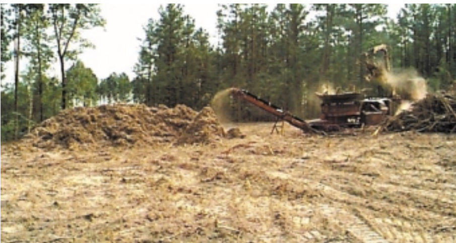
Debris grinding with tub grinder
