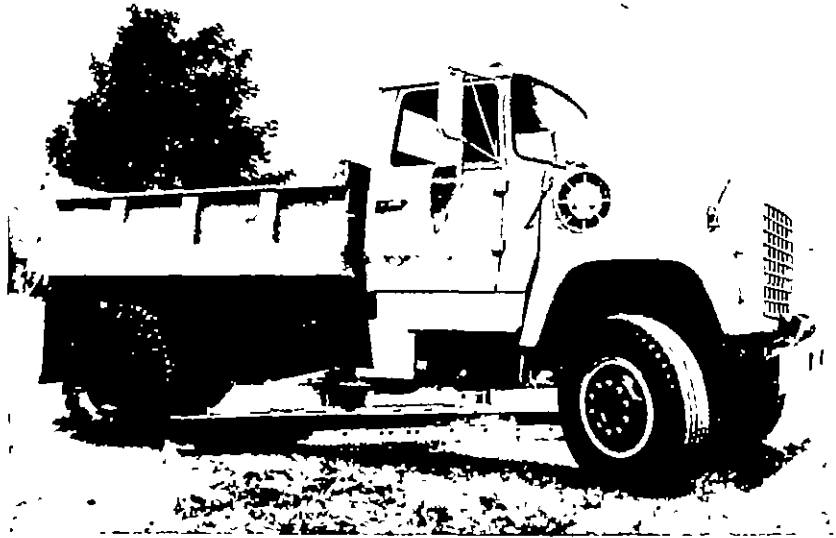
FIGURE 15 FIVE-TON, TWO-AXLE, HEAVY-DUTY TRUCK WITH UNDERBODY SCRAPER
