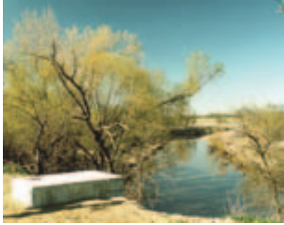
An intake directs water from the Little Arkansas River to the Sedgwick recharge site.
