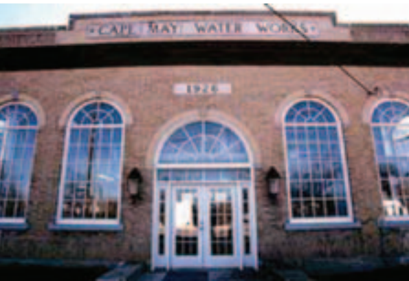
Cape May's desalination plant was built inside the brick building of the former Cape May Water Works.
