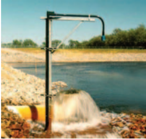
Treated water is being discharged to the Sedwick recharge basin.
