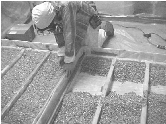
Figure 22: Moving Vermiculite in the Simulated Attic Trusses for Wiring Purposes (perpendicular to trusses)
