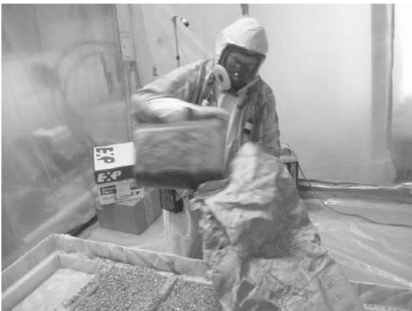
Figure 15: Scooping the Vermiculite Attic Insulation Back to the Product Bags
