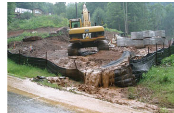
Citizen training programs aim to reduce erosion on construction sites. See page 14.
