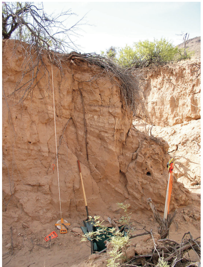
Figure 53. Location of section 4 at Arroyo Grande. The profile height (at location of measuring tape) is approximately 3 m. This stratigraphic section is in a zone of repeated channel incision and filling (note beds that dip steeply to the right of the photo [north, shoreward]); there is therefore little lateral continuity of stratigraphic units at this site.
