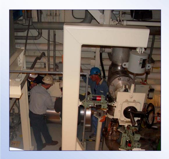
Rigging needs determined through the use of a full scale HPI pump mock-up
