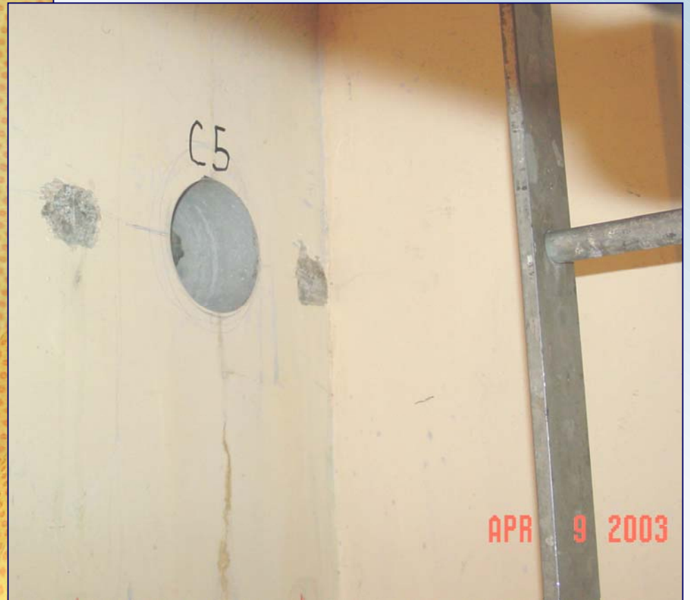
Concrete Core Bore
