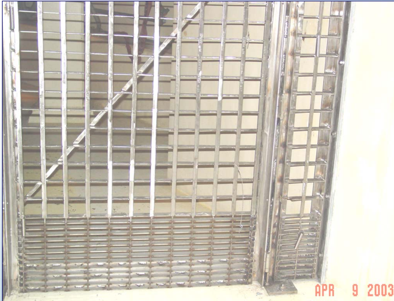
Debris Screen Gate
