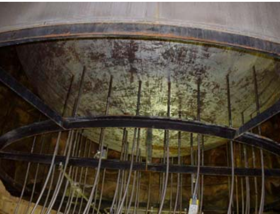
IMI Nozzles at Bottom of Reactor Vessel (Post-cleaning)
