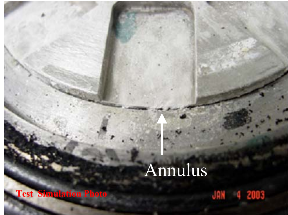
Test #2 (leak rate: 0.0017 gpm) Close-up view of head-to-nozzle annulus showing buildup of white deposits at exit of annulus
