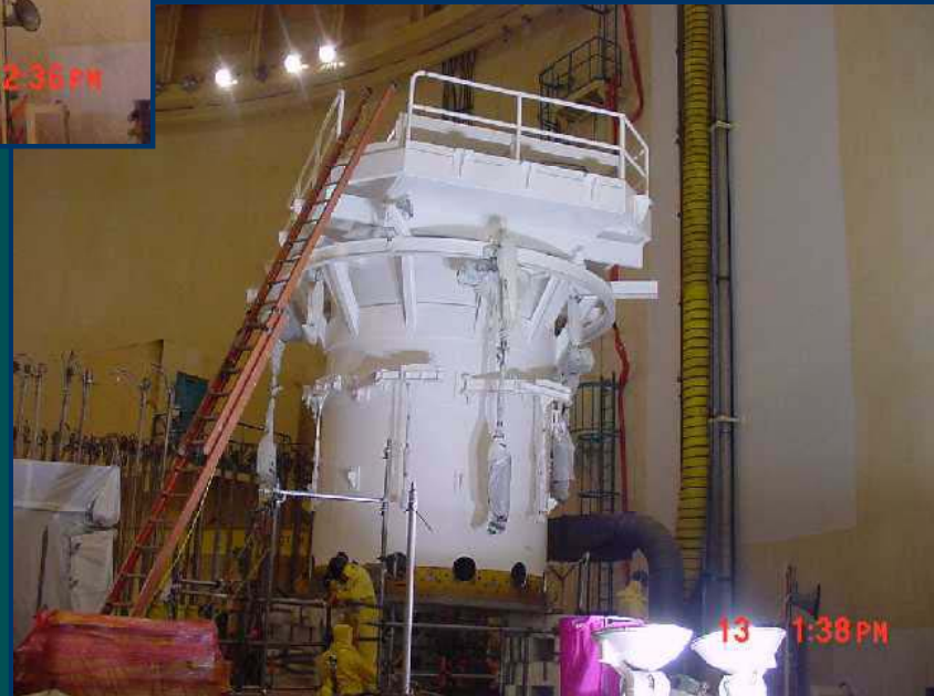
After Sponge Jet-Blasting and Painting
