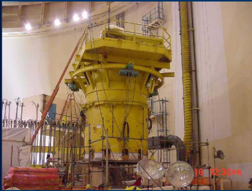
Before Sponge Jet-Blasting and Painting
