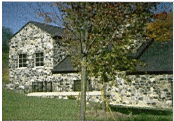
Figure 4.2: Control Building (Birmingham Hills) Retention Basin
