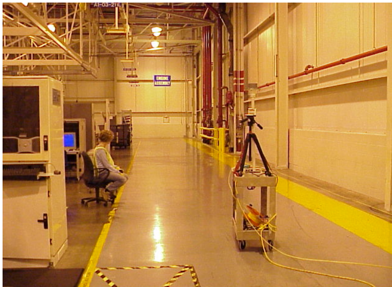
Figure 5-7: Corridor in the engine plant where UWB scattering measurements were made. The receive antenna moved along the corridor on the rolling cart. The VNA and the transmitting antenna were located behind the photographer.
