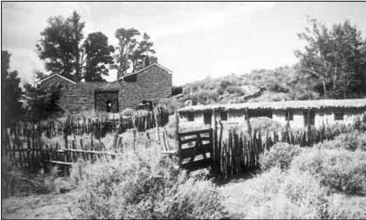
110. Newly re-constructed corral, August 1966 ( Pipe Spring National Monument, neg. 486 ).
