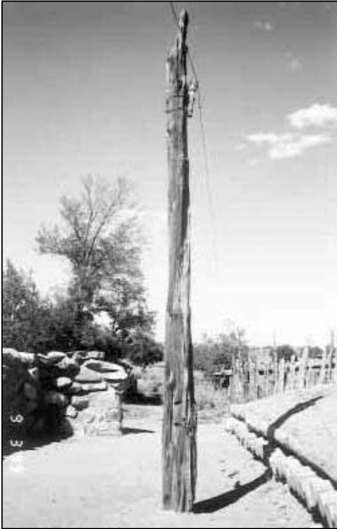
111. An authentic telegraph pole behind east cabin, September 1999
