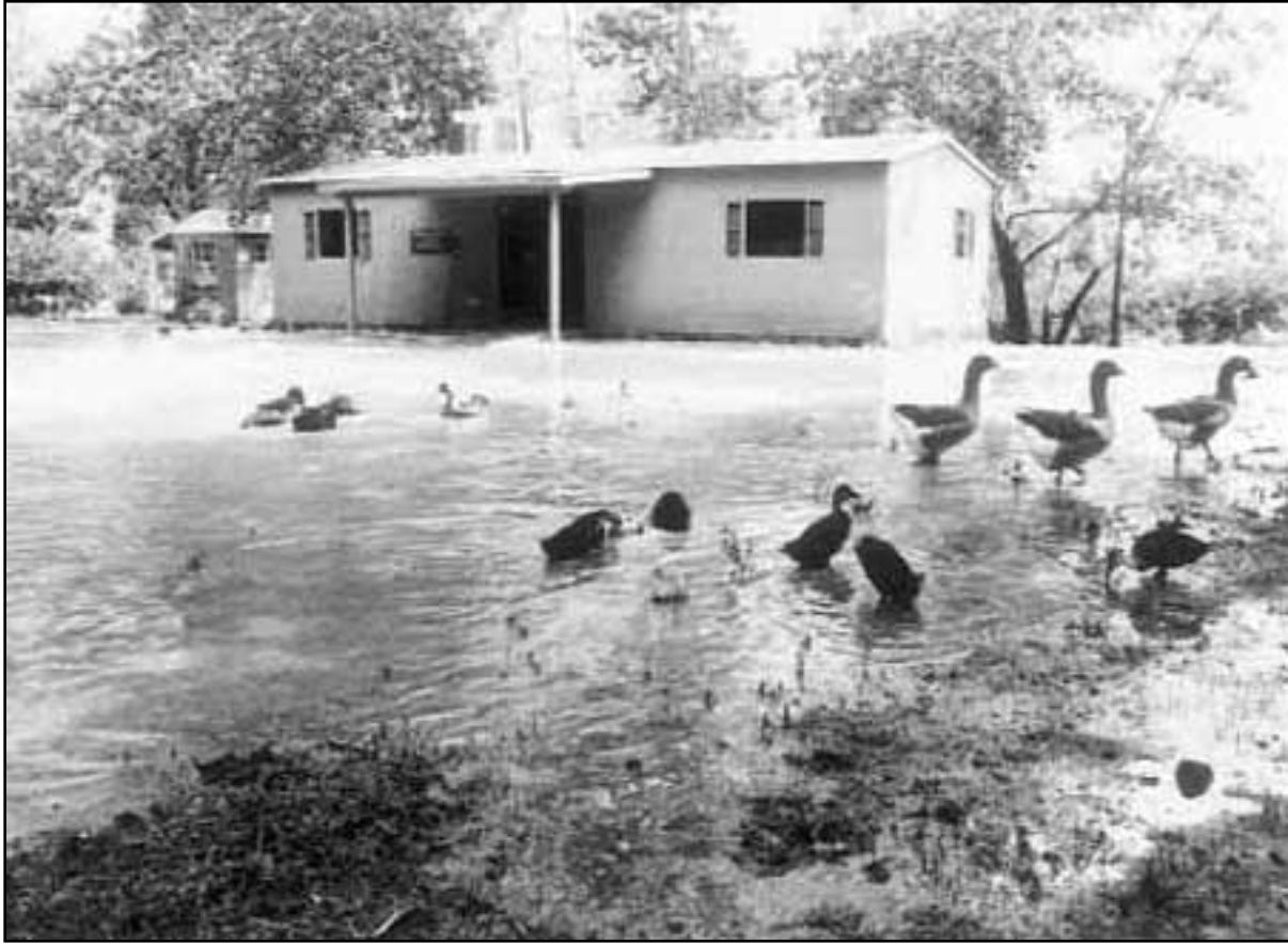
122. Visitor contact station after a flood, August 1969 ( Pipe Spring National Monument ).
