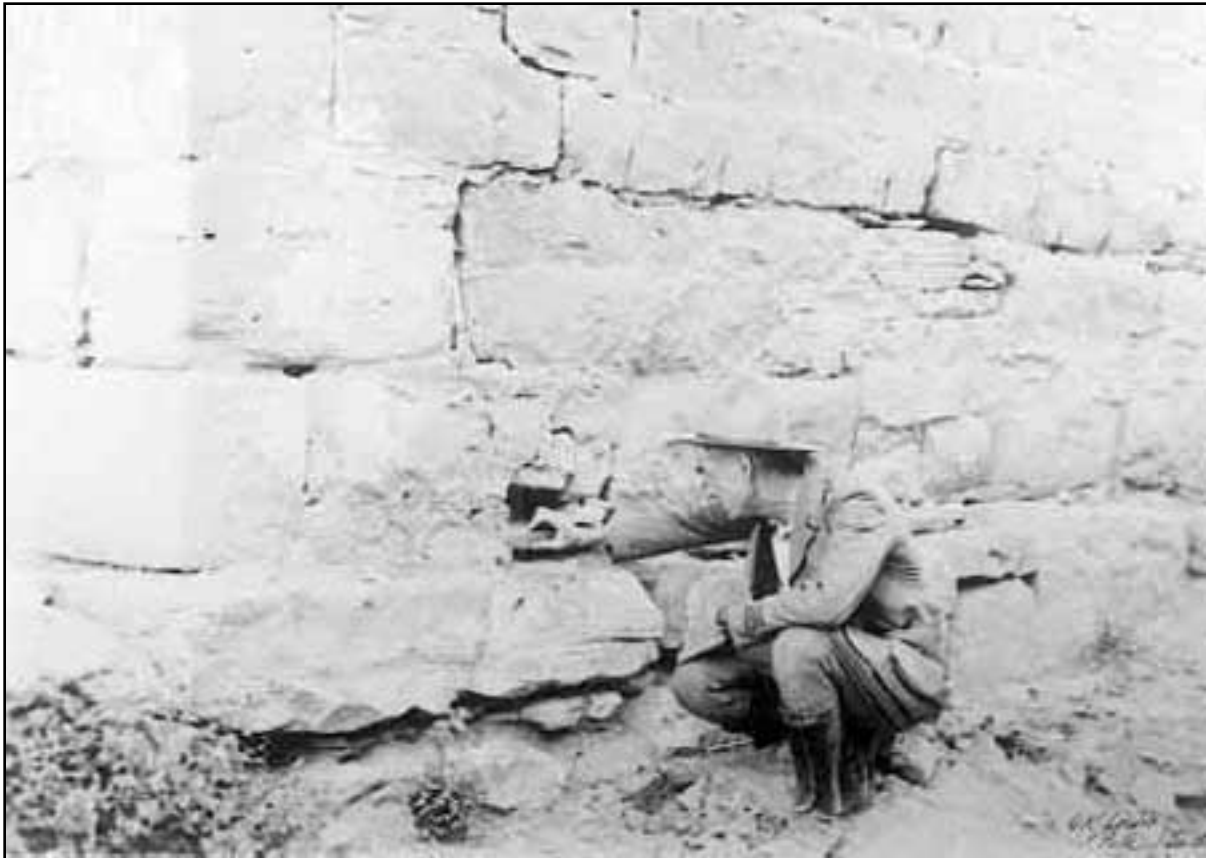
41. Southwestern National Monument's Superintendent Frank Pinkley inspecting southwest corner of fort; undated, ca. 1923-1925 (Pipe Spring National Monument).
