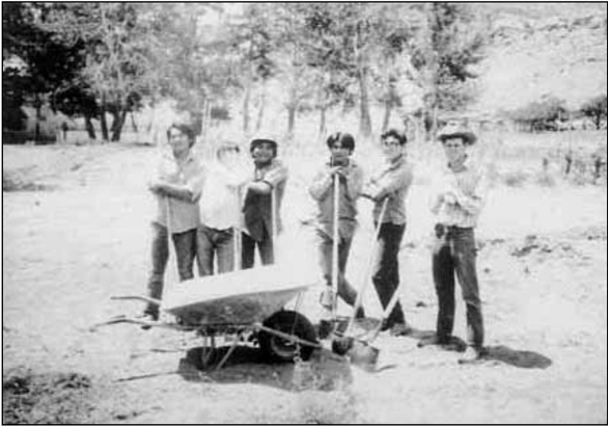
129. NYC crew take a break from work, July 27, 1971.
