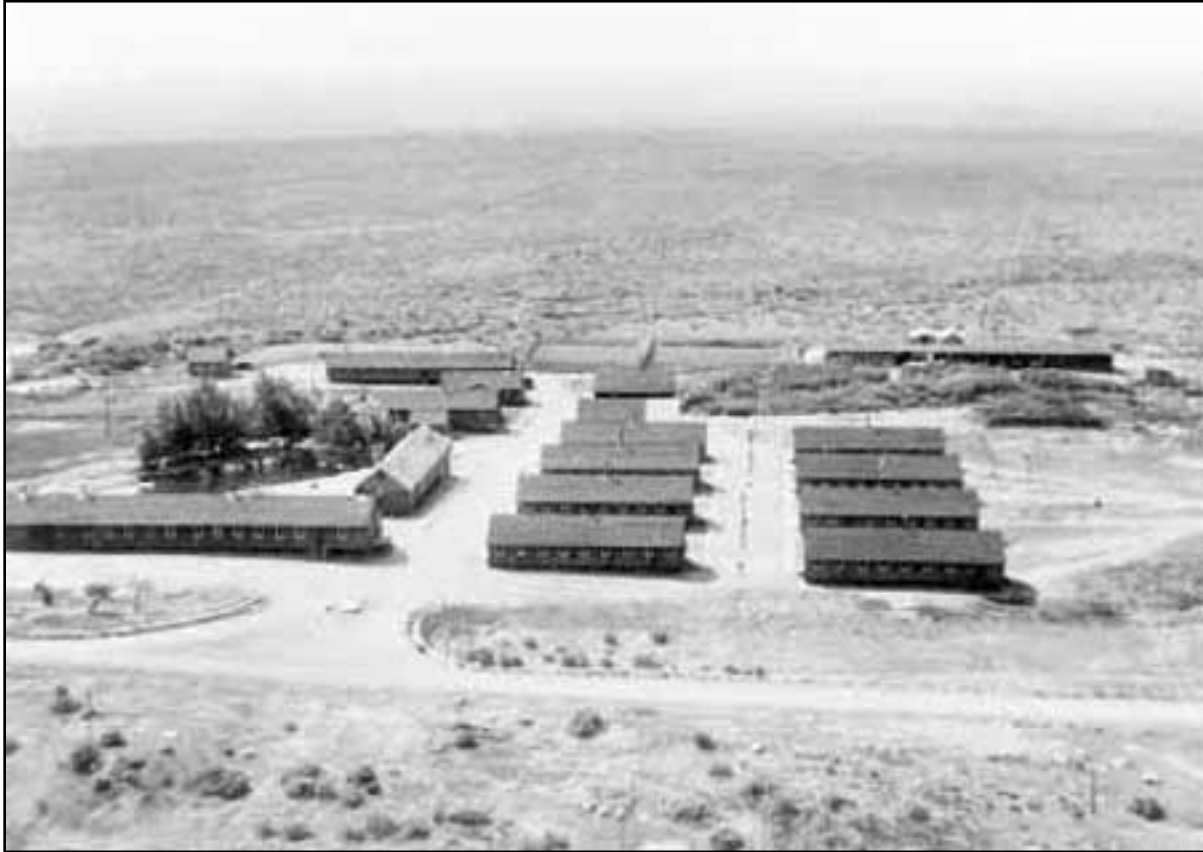
84. View of Camp DG-44, looking south, 1939.
