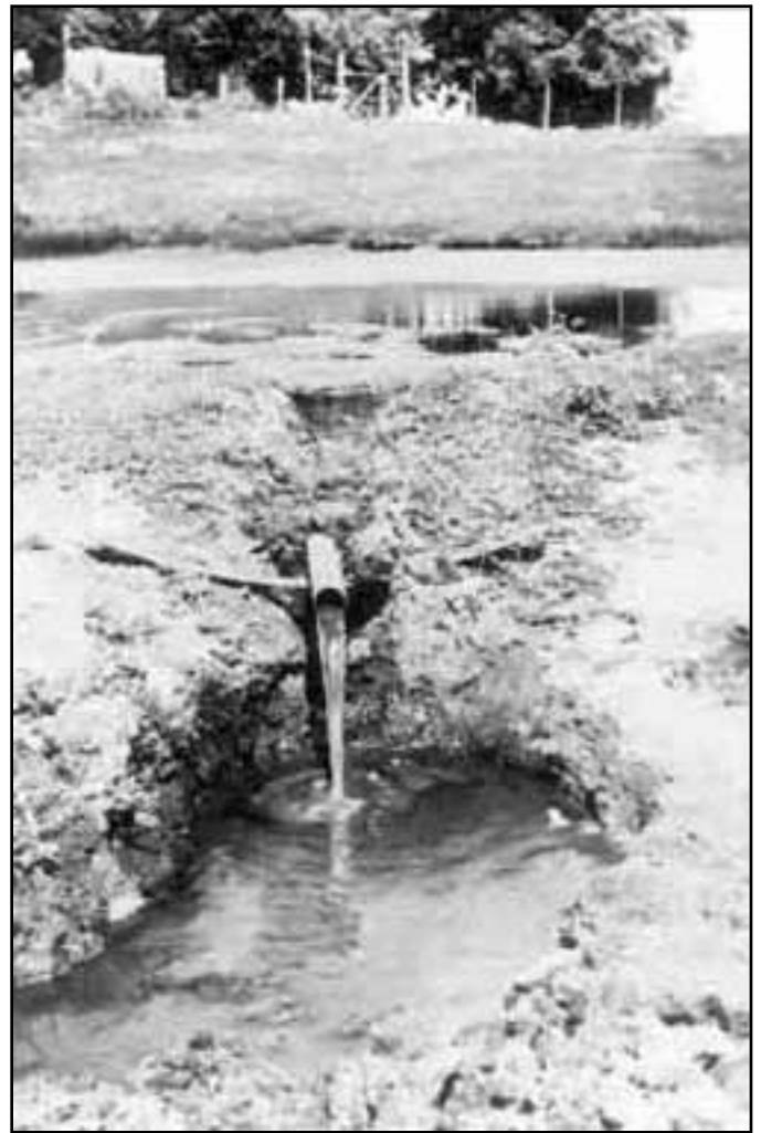
61. Overflow pipe at upper meadow pool, September 1933
