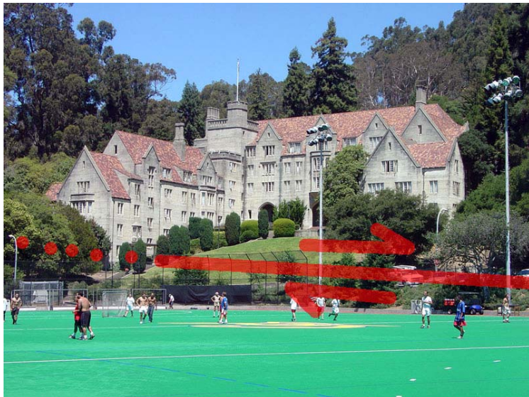
Figure 26. The Hayward Fault crosses the University of California, Berkeley campus. However, with so much construction history there is little visible evidence on the campus itself. In this view, the Hayward Fault is thought to run along the slope just behind Bowles Residence Hall on the southeast side of campus. It grazes the back corner of the building (the library), The California Memorial Stadium is out of view just to the right (south) of this playing field.
