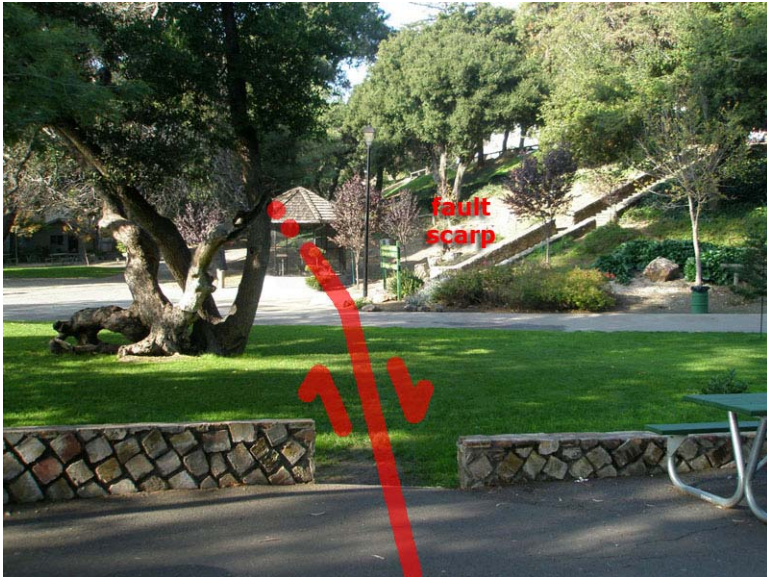
Figure 89. View north past a low stonewall that has been offset by creep along the Hayward Fault (shown in fig. 88). The fault trace is in the path area between the two segments of the wall and continues toward the base of the stairs. The steep slope in the distance beyond the stairway is a fault scarp.
