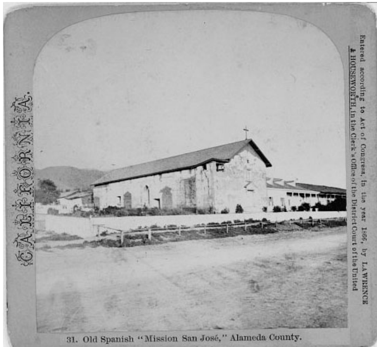
Figure 104. Mission San Jose was founded in 1797. The original church building was constructed of adobe and completed in 1809. The church was nearly completely destroyed by the 1868 earthquake. This historic stereograph of Mission San Jose was taken before the 1868 Hayward earthquake. Photograph by Thomas Houseworth.
