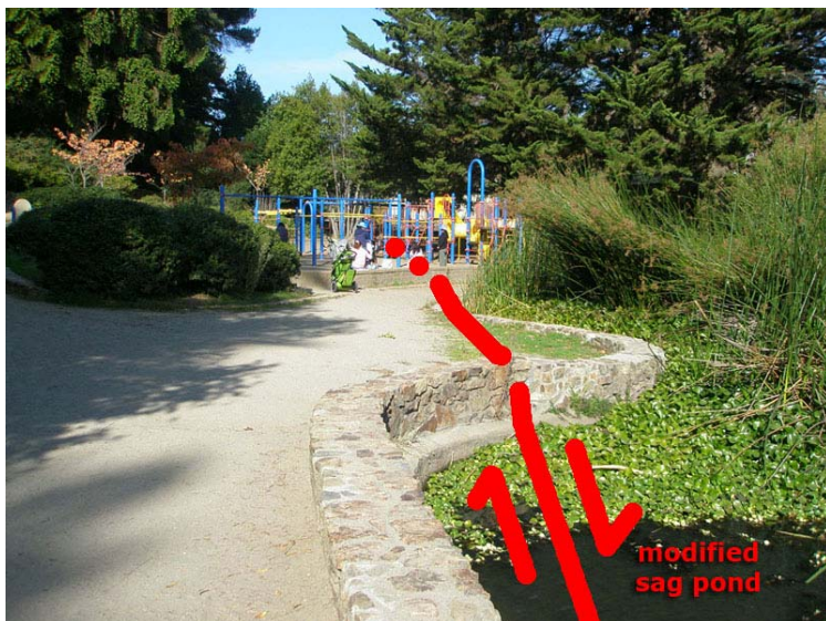
Figure 57. View along an old damaged and repaired wall in the Hayward Fault zone in Monclair Recreation Center (park). Montclair Park's pond is not a sag pond. It was formed artificially around 1910 by the construction of a railroad fill of the Oakland-Antioch line. Passenger service on the rail ended in 1941, and freight service ceased in 1957.
