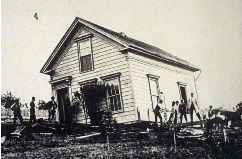
Figure 90. The Pierce's house in Hayward—knocked off its foundation by the 1868 earthquake. Image courtesy of the Bancroft Library, University of California, Berkeley.
