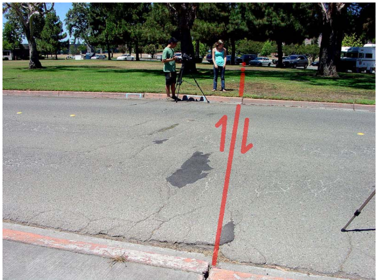
Figure 96. The Hayward Fault crosses through Fremont's Central Park. This view shows two USGS interns photographing offset curbs and fractures where the fault crosses Sailway Drive on the west shore of Lake Elisabeth. Look for the offset curbs and fractures in the pavement about 200 feet east of the intersection of Sailway Drive and Paseo Padre Parkway.
