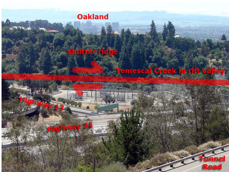
Figure 45. View southwest across Highway 24 toward the PG&E Claremont Substation near Lake Temescal. The tree-covered slope beyond the electrical power station is on the west side of the Hayward Fault rift valley incised by Temescal Creek. Downtown Oakland is in the distance. The tree-covered ridge is a shutter ridge ("shutting in" and diverting Temescal Creek). Lake Temescal is to the right of this view taken from Tunnel Road, north of Highway 24. The neighborhood of Buena Vista is built on the shutter ridge west of the Hayward Fault rift valley.
