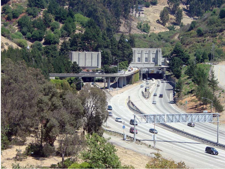
Figure 46. View of the western portal of the Caldecott Tunnel on Highway 24. The Caldecott Tunnel cuts through the Berkeley Hills. Construction of the tunnel began in 1929, and the first two tunnel bores were completed in 1937; a third bore was completed in 1964. An additional bore has been approved for construction. The western portal of the Caldecott Tunnel is located in Claremont Canyon, about one mile upstream from Lake Temescal. The forested ridge above the tunnel is mostly within the Robert Sibley Regional Preserve.
