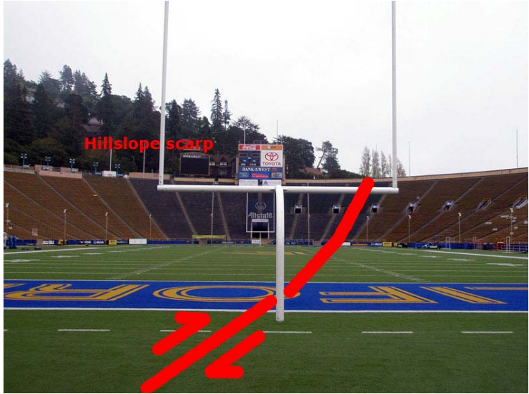
Figure 27. View looking south past the goal post near the north end of California Memorial Stadium. Beyond the stadium, the Hayward Fault continues south along the base of a slope into residential neighborhoods of Berkeley. In the stadium, the fault runs through the playing field and through the section of seats (section KK) in the distance to the right of the goal post.
