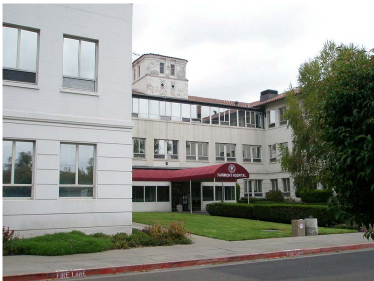
Figure 74. Fairmont Hospital is an Alameda County facility in San Leandro. Some of the original hospital buildings were constructed on the Hayward Fault but were later abandoned or modified. Evidence of the active creep of the fault can be seen on the hospital grounds in the form of cracks in the pavement and older walls and offset curbs, particularly on the east and south sides of the main hospital building.
