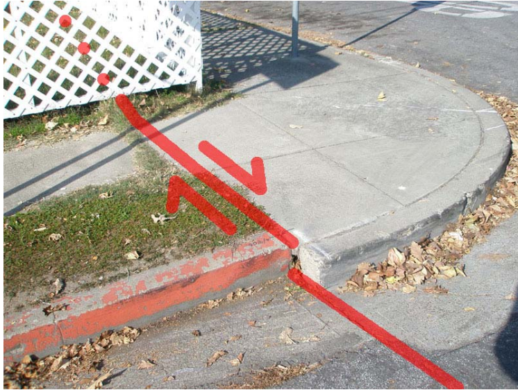
Figure 78. View of an offset curb at the southwest corner of Prospect Street and Rose Street north of downtown Hayward. The displacement of the curb is consistent with the relative right-lateral displacement of the Hayward Fault. A right-lateral displacement refers to the relative motion of the two sides of a strike-slip fault . Offset features along the Hayward Fault show that the west side is moving northward relative to the east side of the fault.
