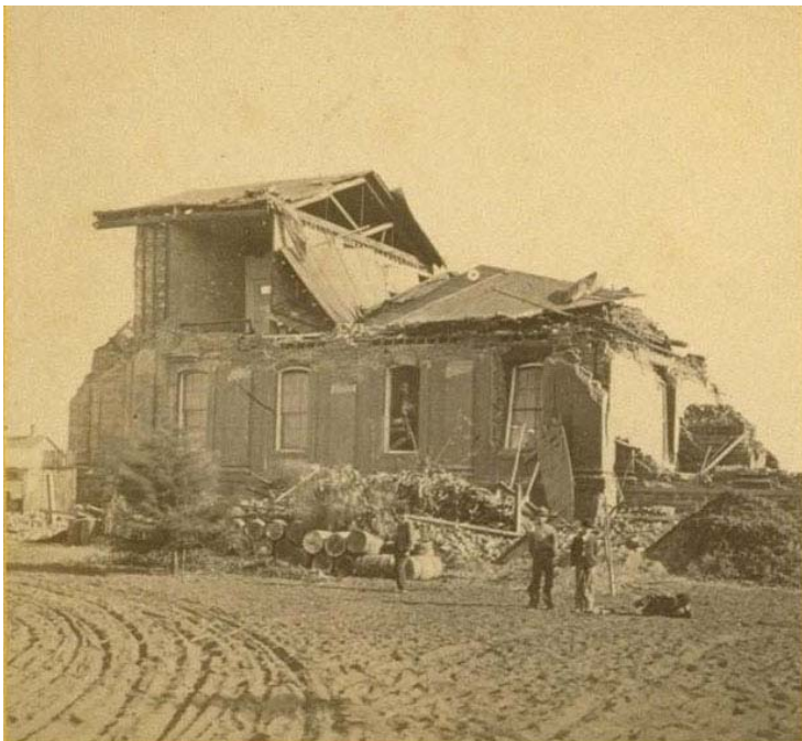
Figure 70. Historic photograph by Carleton Watkins showing the condition of the Alameda County Courthouse after the 1868 Hayward earthquake. One person was killed when the courthouse collapsed. Note that the building on the far left appeared to escape damage and still had its chimney. The old courthouse was located at the intersection of Davis and Clarke Streets.
