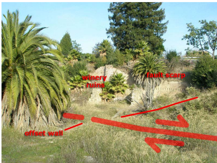
Figure 108. This view is looking east at the property owned by BART near Osgood and Washington in Fremont. The photo shows the ruins of the Gallegos (Palmdale) Winery, which was built into a hillside that is a fault scarp of the Hayward Fault. In the brush-covered field is a stone perimeter wall built in 1884. By 1985, this stone wall had been offset by 2.5 feet of accumulated right-lateral creep on the main trace of the Hayward Fault (Lienkaemper, 2006).
