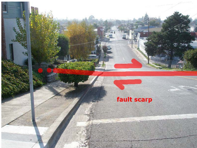
Figure 80. View west along Simon Street from the intersection of Prospect Street in Hayward (Mission Boulevard is in the distance). The slope in the foreground is a scarp of the Hayward Fault. The active trace of the fault crosses the street where the street curb (on the left side of the street) shows displacement from creep.
