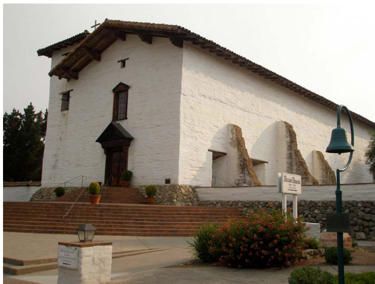
Figure 105. A new church constructed of wood was built on the rock foundation of the old church. However, the wooden building was moved and the San Jose Mission church was rebuilt (restored) to look like the original; construction was completed in 1985. The mission is still used for religious services and has a unique historical collection of artifacts in a museum in one of the remaining original adobe buildings next door that survived the 1868 earthquake.
