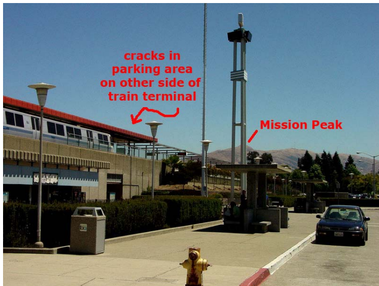
Figure 94. The Fremont BART station is the current terminus of the rail line. The track ends a very short distance from the Hayward Fault. Cracks in the pavement caused by slow creep of the fault can be seen in the train parking area on the southeast side of the train station. This view is looking southeast at the BART station with Mission Peak in the distance.
