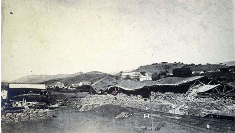
Figure 91. Edminton Grain Warehouse and flour mill—collapsed during the 1868 earthquake. The hills in the distance are the fault scarp/shutterraidge of the Hayward Fault along Prospect Street between Hotel Avenue and Rose Street on the south side of downtown Hayward. Image courtesy of the Bancroft Library, University of California, Berkeley.
