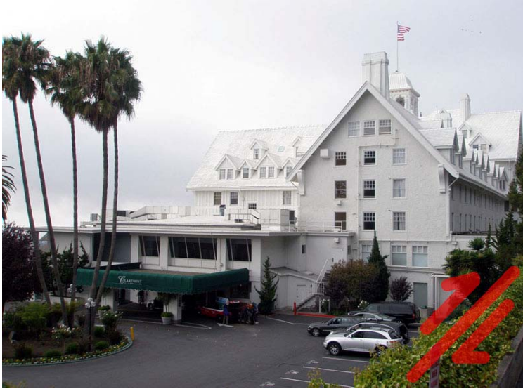
Figure 36. The Hayward Fault runs through the parking lot and beneath the corner of the building (on the right side of the photograph) near the south entrance to the Claremont Hotel.
