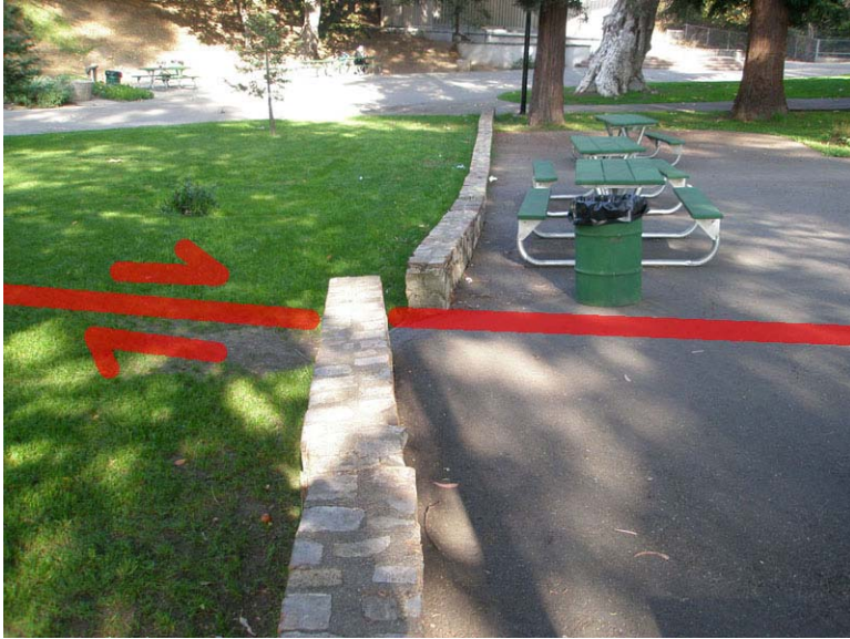
Figure 88. This old, low stonewall in Memorial Park near downtown Hayward has been displaced by creep along the Hayward Fault. This view is looking east.
