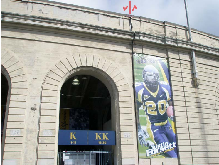
Figure 30. View of the offset outer wall on the south side of Berkeley Memorial Stadium in section KK where damage to the stadium by the creeping Hayward Fault is most obvious.
