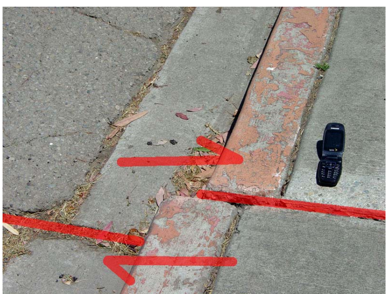
Figure 97. Close-up view of an offset curb on Sailway Drive in Fremont Central Park (in the same location as fig. 98).
