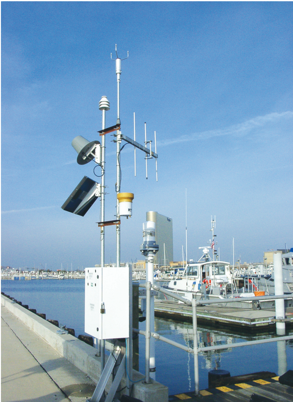
Figure 2. USGS tide gage/weather station at Absecon Channel in Atlantic City, NJ, which transmits tide-level and meteorologic data.
