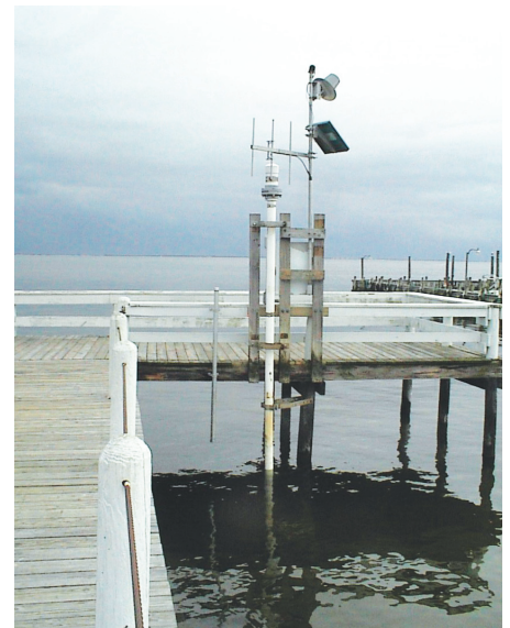
Figure 4. USGS tide gage at Barnegat Bay in Waretown, NJ, which transmits tide-level data.
