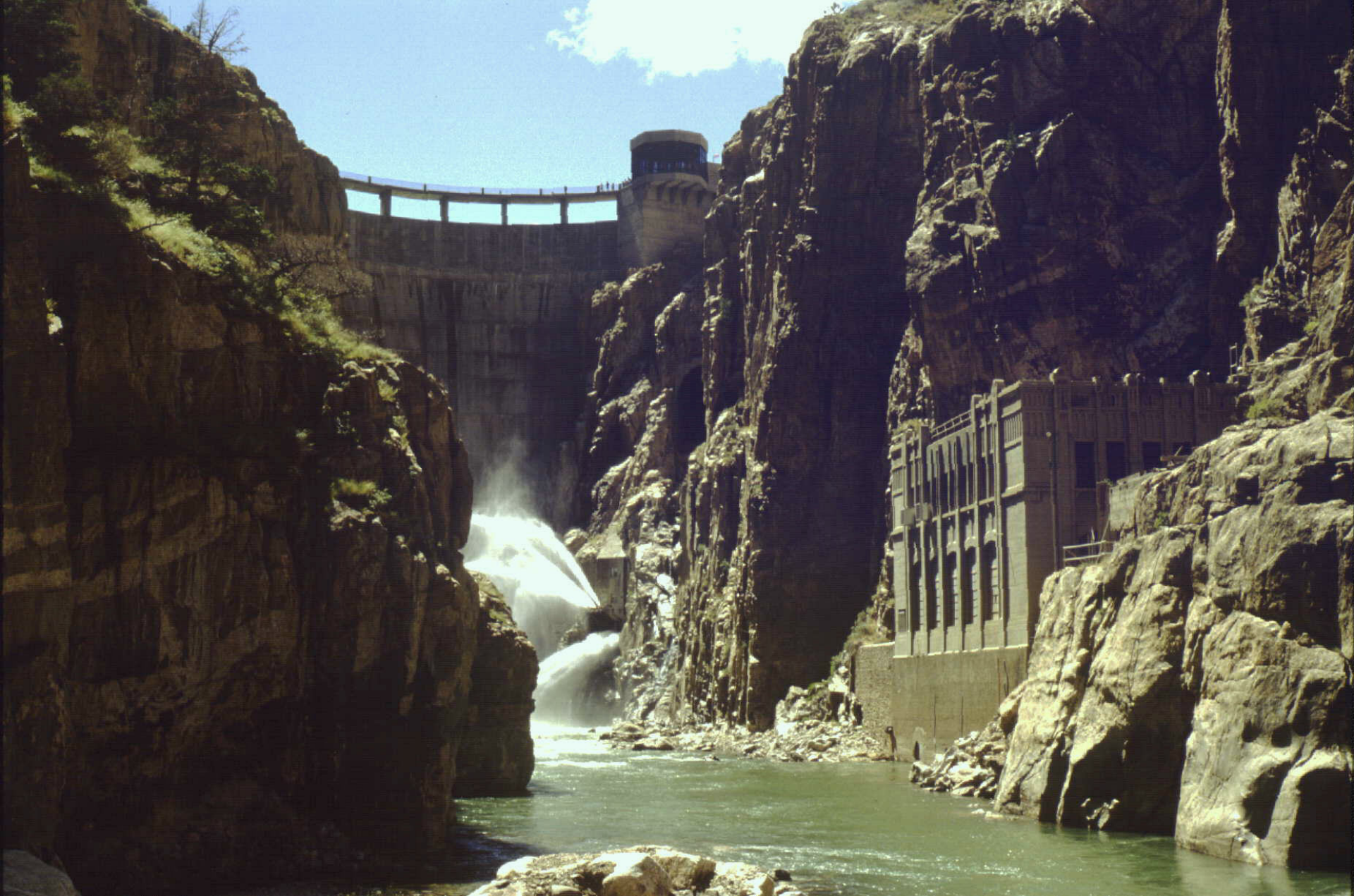
Buffalo Bill Dam, Visitor Center, & Shoshone Powerplant
