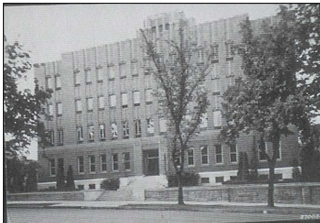
Forest Service Building, 25th and Adams, Ogden, Utah
