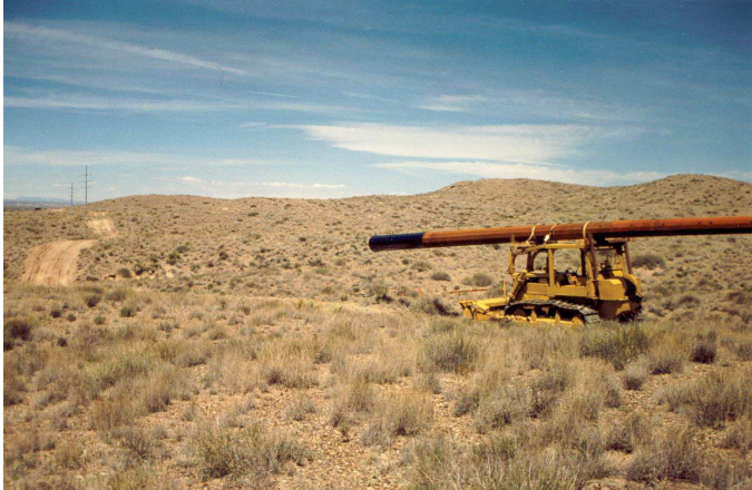
Bulldozer hauling a structure
