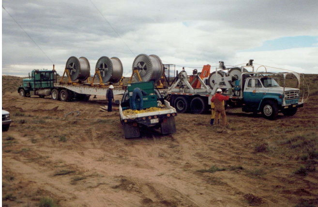
Pulling trailer and utility truck
