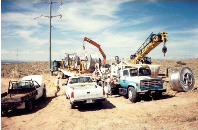
Pulling trailer and pick-up trucks
