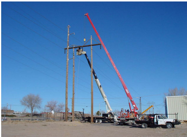
Crane and Bucket Truck
