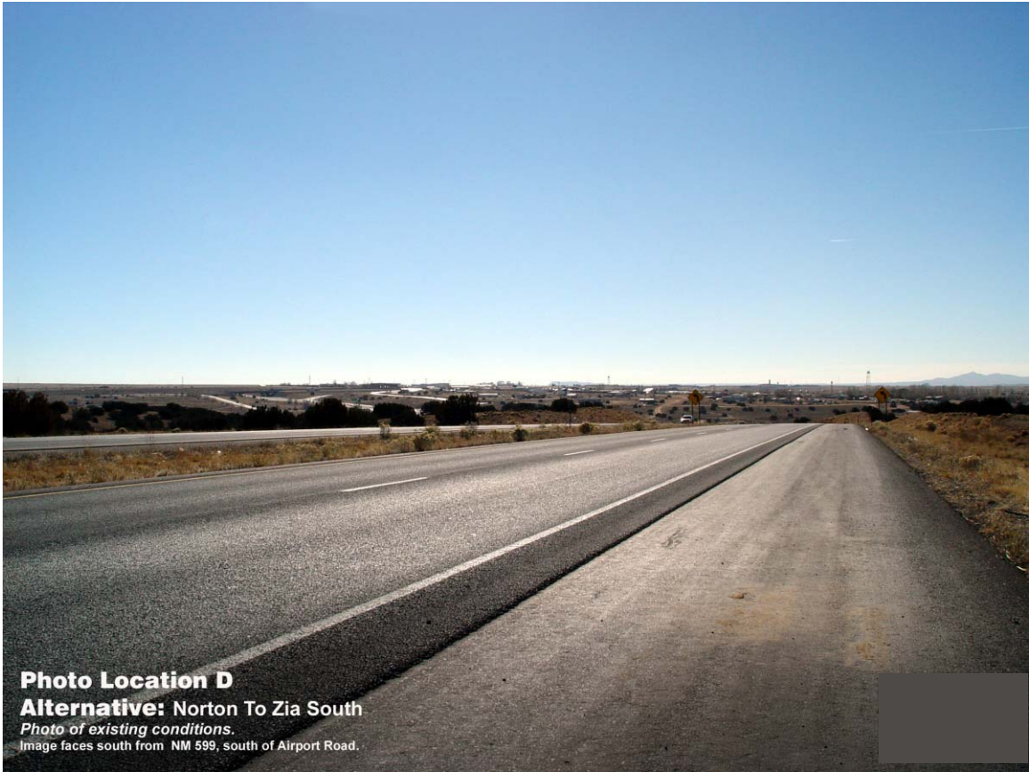
(From new line portion)
