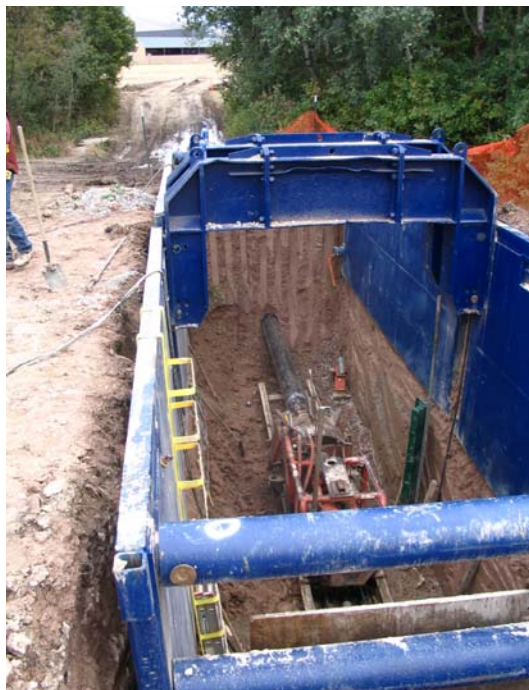
Water Line Construction Under Butler Creek
