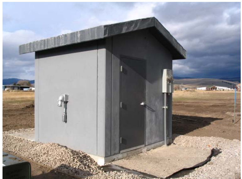
Sewer Lift Station — Concrete Pad to be Poured
