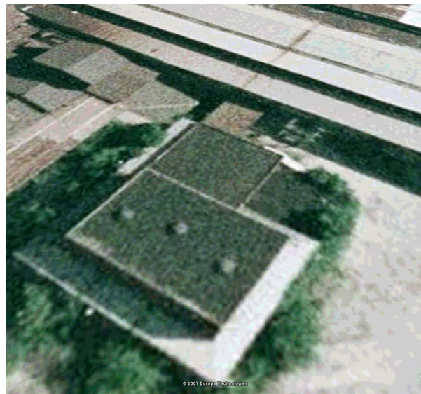
Figure 4. Aerial View of New Betatron Building (Google 2007)
