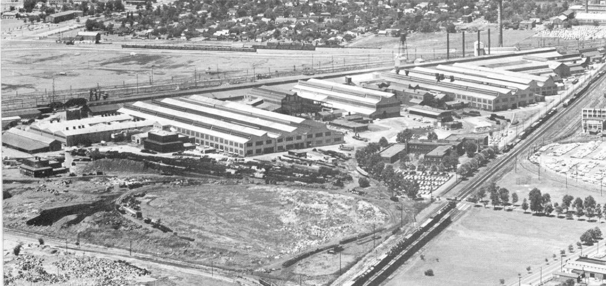
Figure 1. Aerial View of General Steel Castings Division in Granite City (GSI n.d.)
