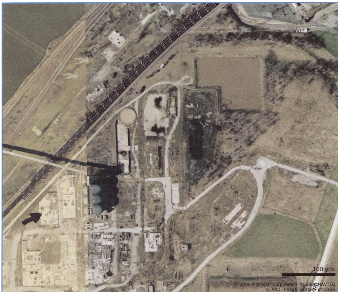
Figure 2-1: Aerial Photo of Blockson Chemical Company Site, Building 55 marked with Arrow
