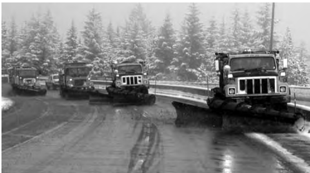
ODOT plows clear the road at Siskiyou Summit. The agency spends more than $3 million on statewide snow removal operations each year.
