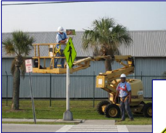
Warning sign has yellow ultra-bright LEDs that blink up to 60 times per minute.
