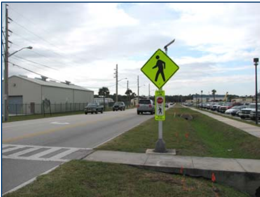
Pedestrian crossing sign and its flashing LED lights are clearly visible to approaching vehicles
