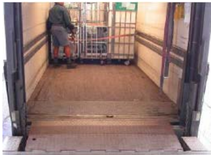
New loading dock ramps are hydraulically controlled eliminating need to manually move dock boards.
