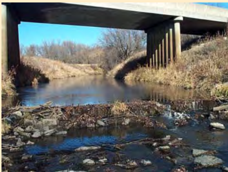
Before Fish Passage Improvement
