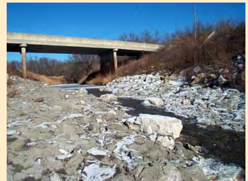
After Fish Passage Improvement
