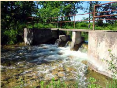
Before Fish Passage Improvement
