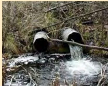
Before Fish Passage Improvement Johnson's Crossing culvert replacement in Michigan. This project reduced sediment loading and enhanced fish passage for brook trout.
