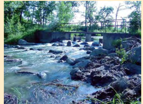
After Fish Passage Improvement
