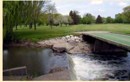
Before Fish Passage Improvement
