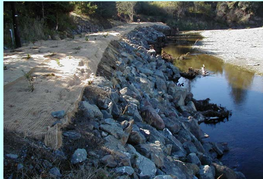
After installation of wood.
