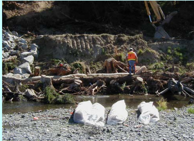
Cross log locks into stumps to prevent washout.
