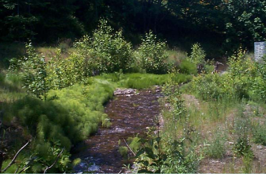
Stream channel prior to construction. notice the standpipe in the upper right.
