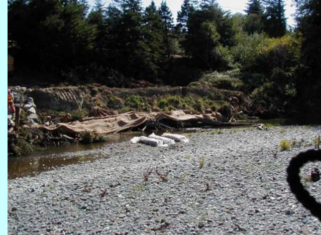
Biodegradable fabric secured to log.
