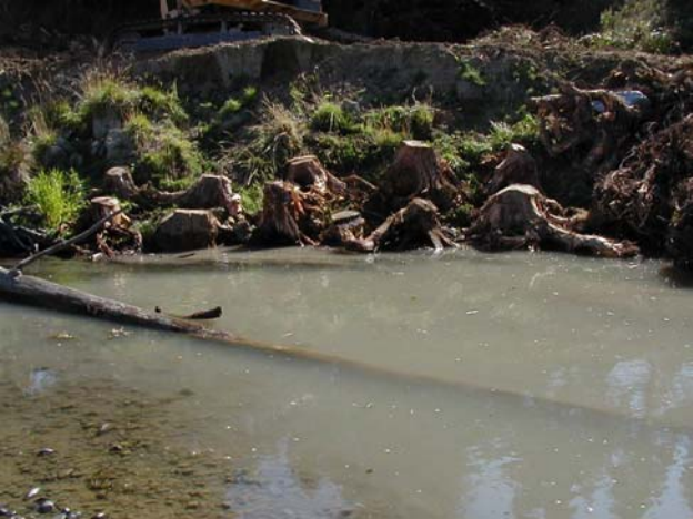
Installation on stumps for bank footing stability.
