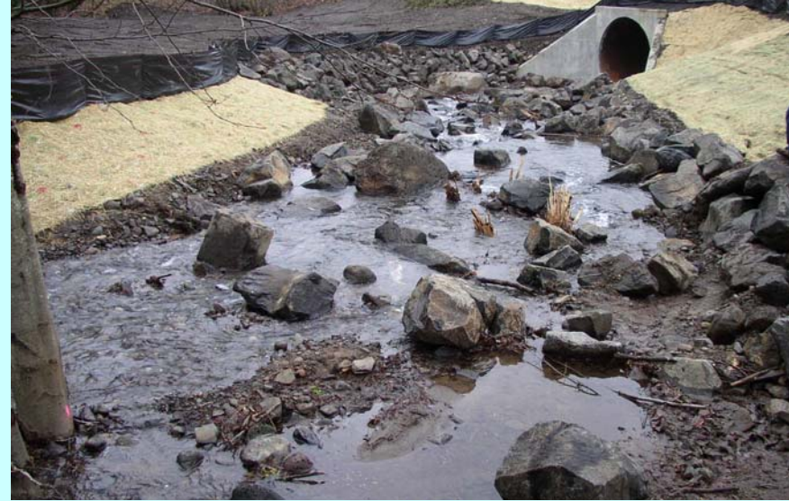
New channel after construction with bank slopes are seeded with matting.
