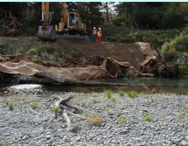
Re-sloping bank to 2:1 for stability.
