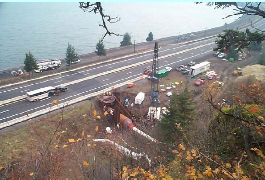
There is very minimal traffic disturbance during installation.
