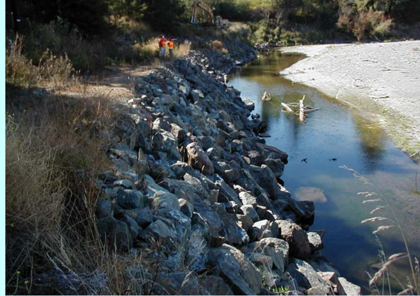
Bank Prior to installation of wood.
