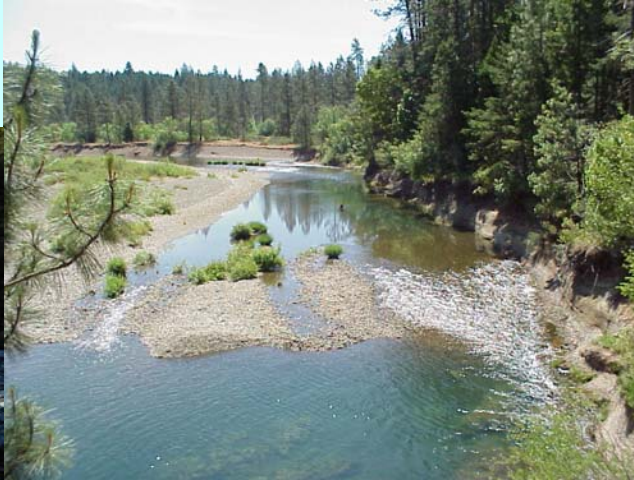
Prior to installation of Rock Barbs the river was moving to the south.
