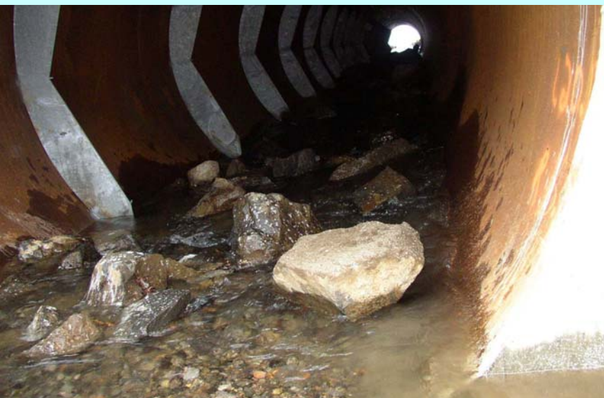
7% slope, simulated streambed with side baffles, heavy bedload movement.
