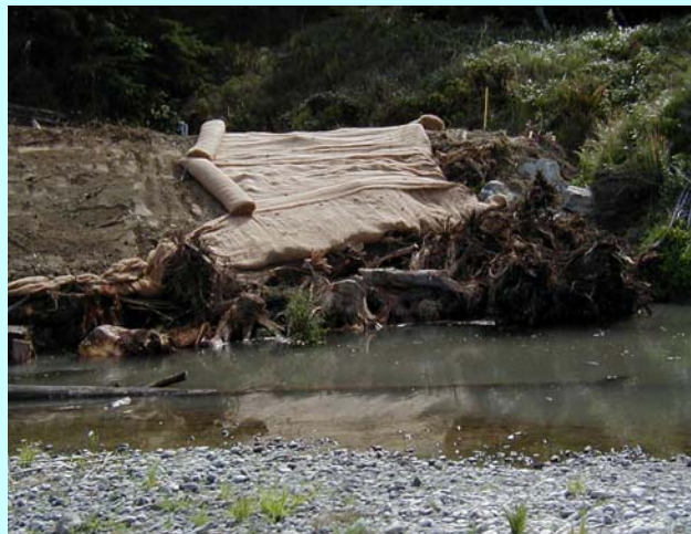
Fabric laid over seeded soil.
