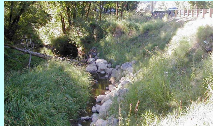
August 14th, 2000, 10 months after installation there is abundant vegetation growth.
