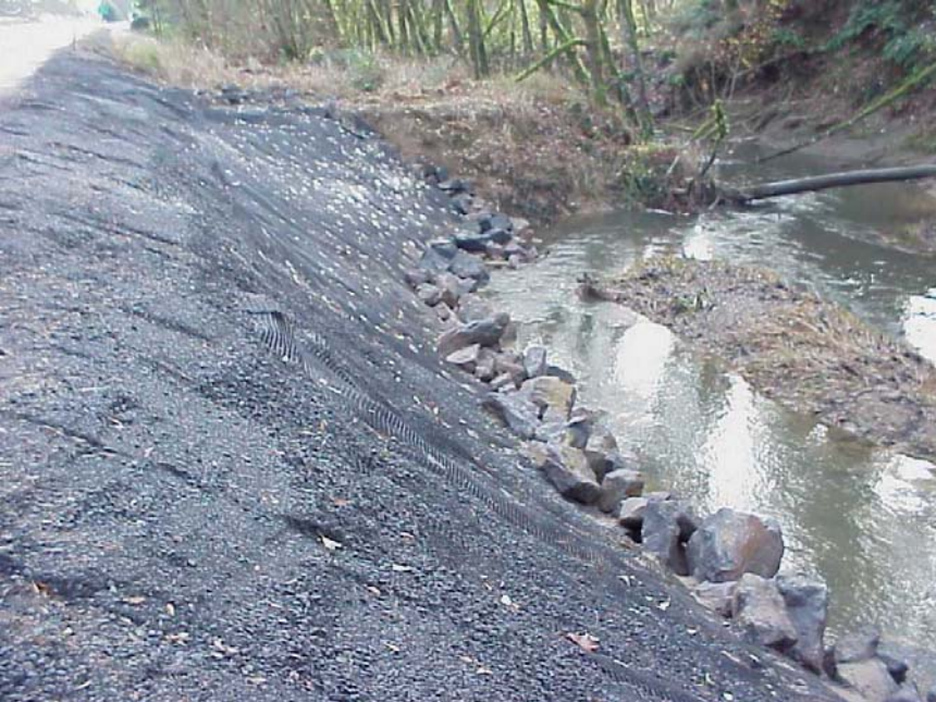
Nov. 30th 1999, just after installation.
