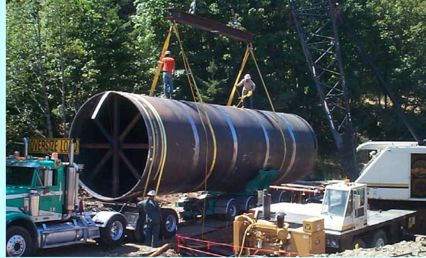
Delivery of a section with bracing to retain shape during transport.
