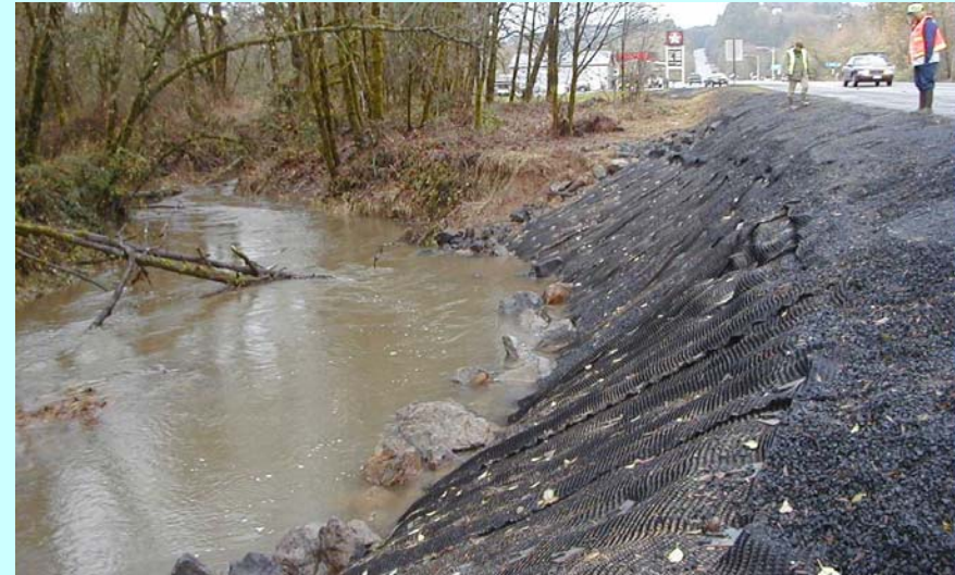
December 6th, 1999, Pyramat and riprap holding well.
