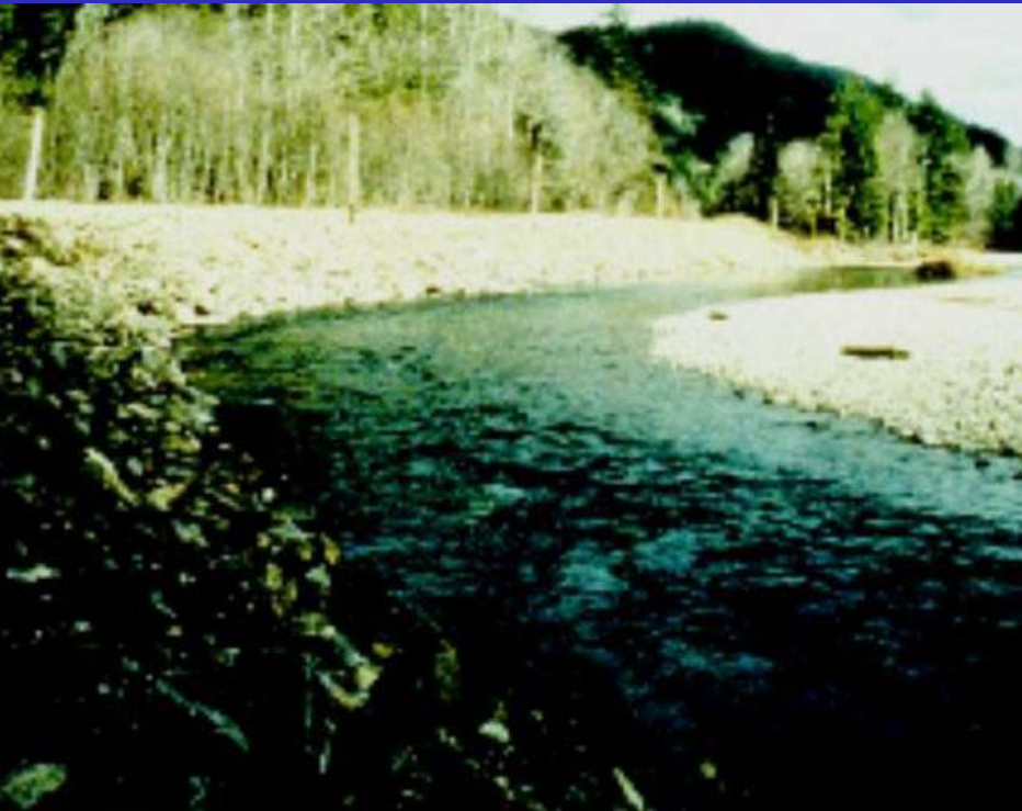
Traditional Streambank Protection
