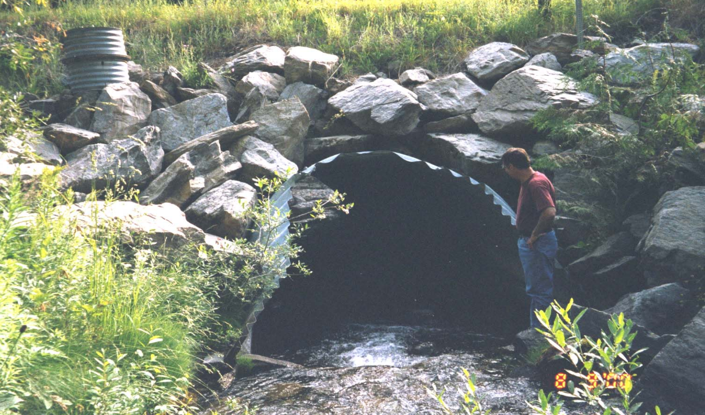
NFLJ, CULVERT INLET, 2000.
