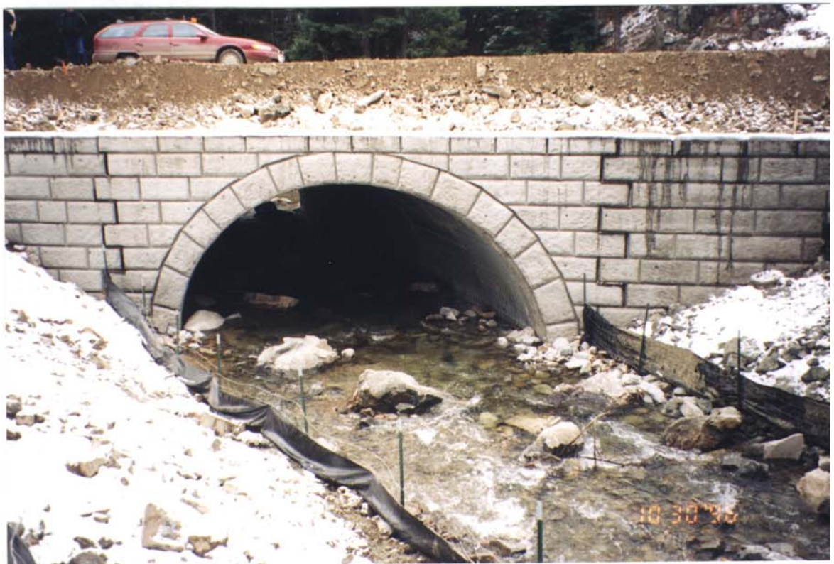
NORTH FORK SALMON RIVER, IDAHO. 1996. STA 17±, OUTLET (UPPER), INLET (LOWER)
