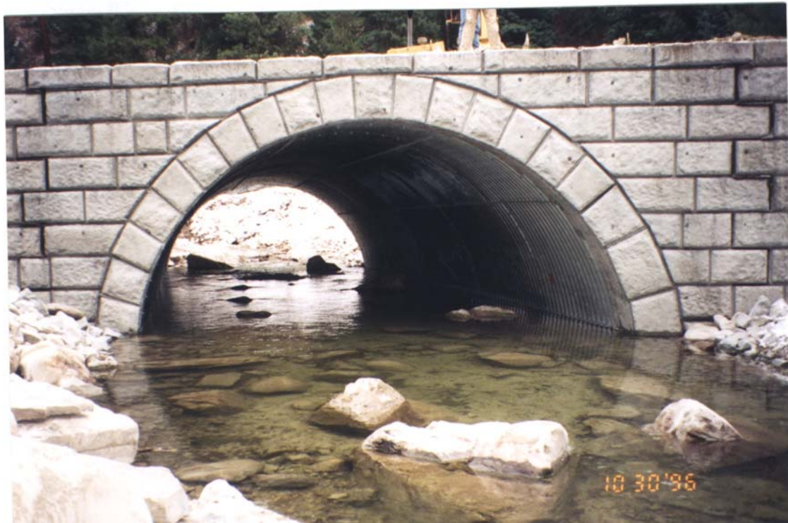
NORTH FORK SALMON RIVER, IDAHO. 1996. STA 28±, INLET (UPPER), OUTLET (LOWER)
