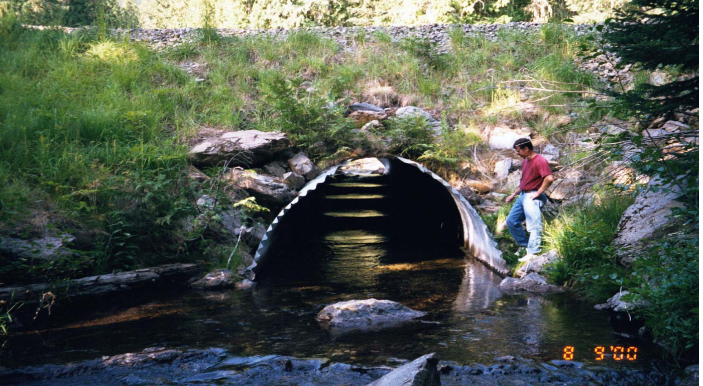
NFLJ, CULVERT OUTLET, 2000.
