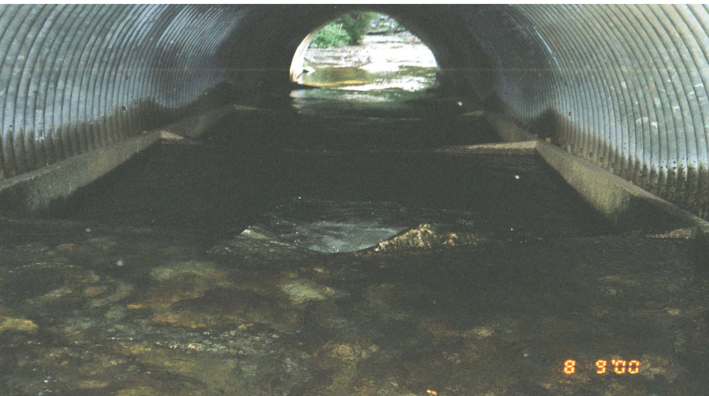
NFLJ, CULVERT BARREL, 2000. FACING D/S.
