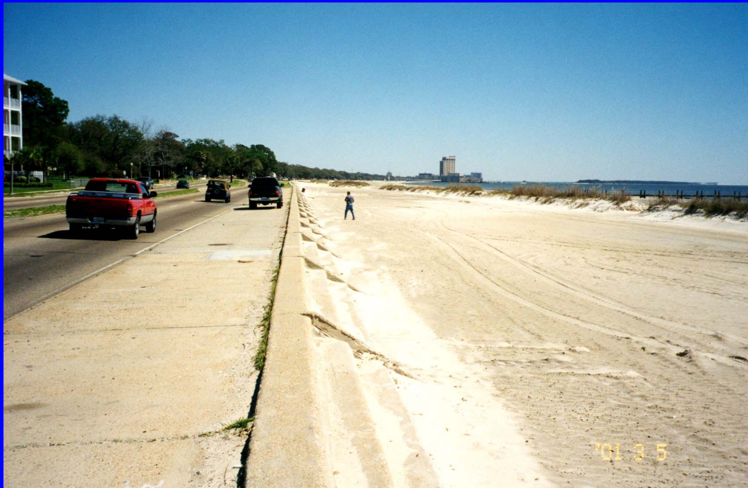
Beach nourishment and stepped seawall US Highway 90, Biloxi, Mississippi
