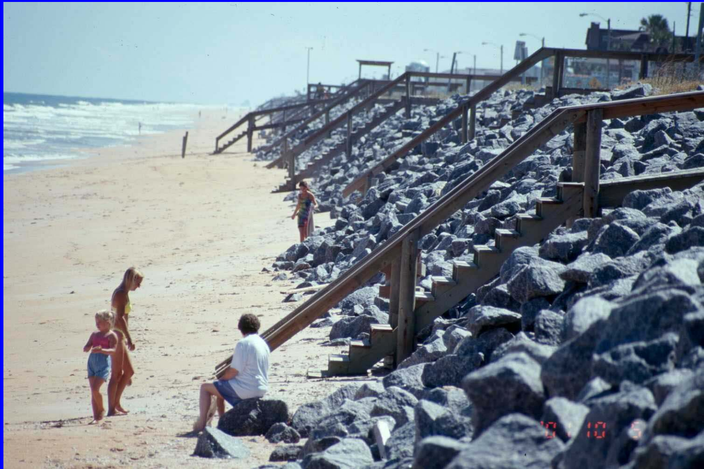
Florida Highway A1A revetment Flagler Beach
