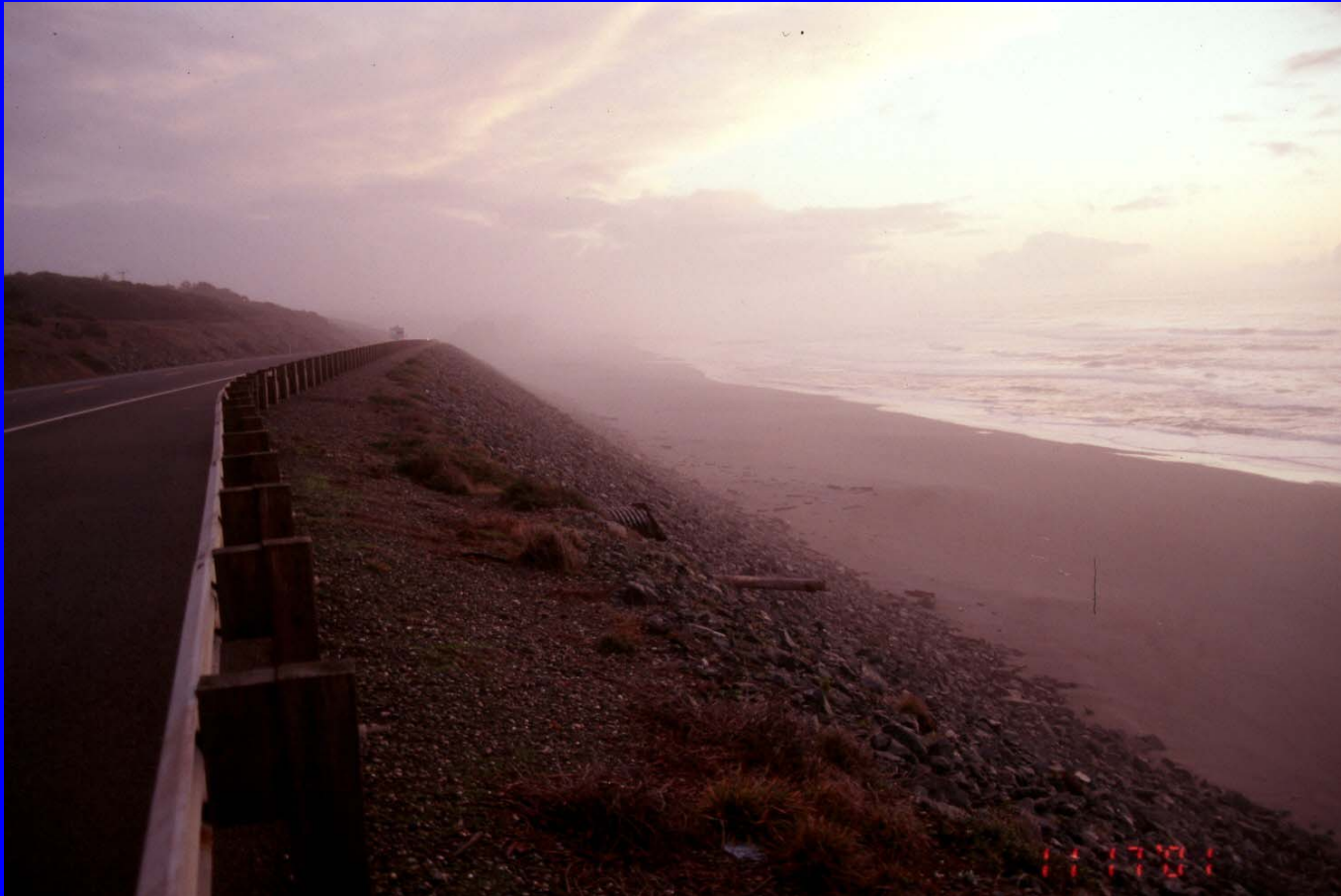
U.S. Highway 101 revetment Curry County, OR
