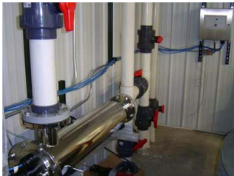
-USFWS The new ultraviolet unit at the Genoa National Fish Hatchery will be used to sterilize lake sturgeon culture water.
