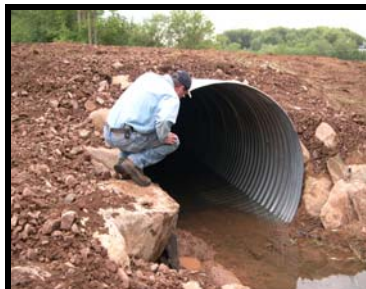
Newly installed culvert on Little Whittlesey Creek.
