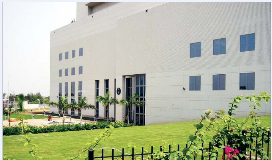
The new U.S. Embassy Compound, Abuja, Nigeria State Department Photo
