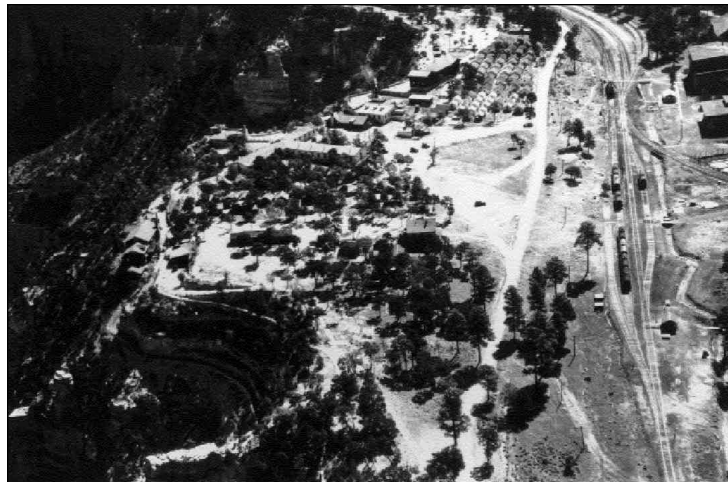
Figure 16. Aerial view of the South Rim, facing east, 1932. Kolb Studio is at center left, the Brown Building and Bright Angel Hotel tent cabins at center top and the post office (former Cannon Hotel) in the center. This photograph was taken three years before demolition of the Bright Angel Hotel and tent cabins, construction of the Bright Angel Lodge and wood-frame cabins, and reconstruction of the Hermit Rim Road. The power house laundry building, and wastewater settling ponds are visible at upper right. GRCA 9543; Fred Harvey Company photo
