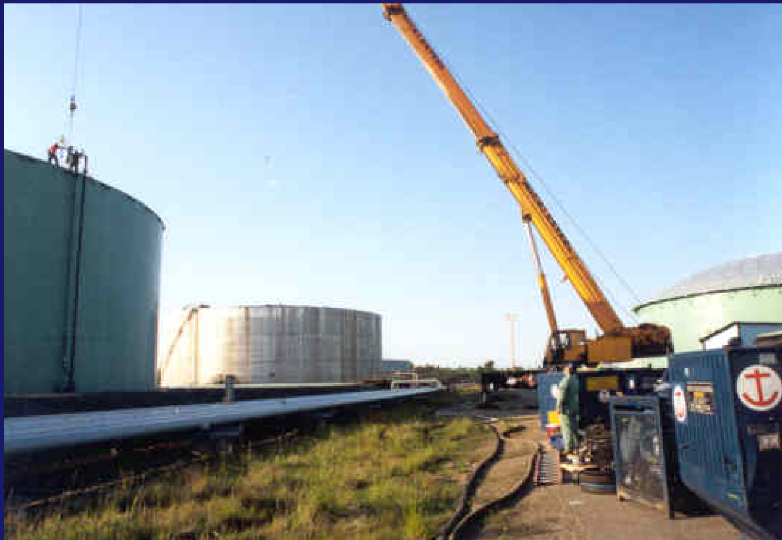
Floating Roof Mechanical Failure - Bellingham, Washington - 2000
