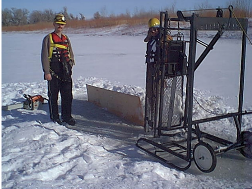
Figure 7. Slot cut with the JSG and ¼” plywood inserted in slot.
