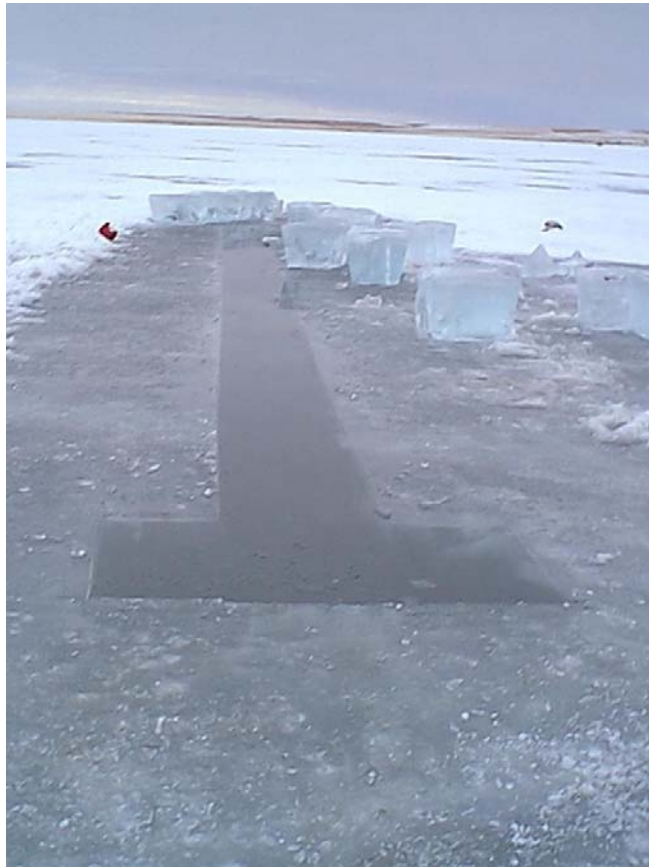
Figure 2. Slot with Recovery Sump (Approximately 50 Feet long)
