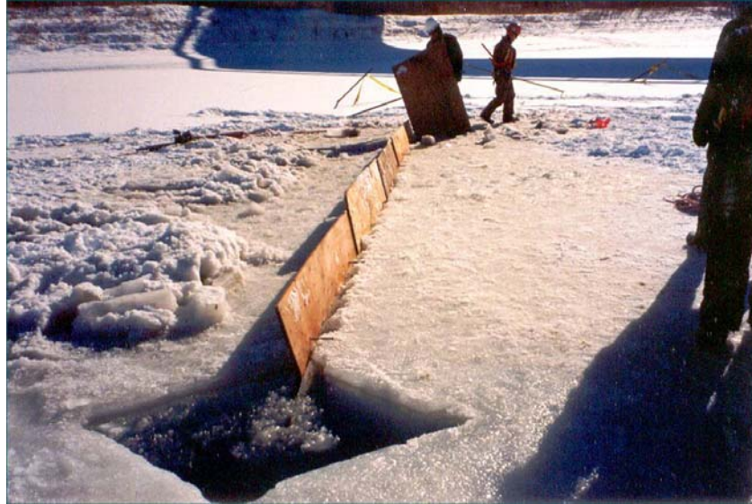
Figure 3. Diversionary Plywood Barrier Method
