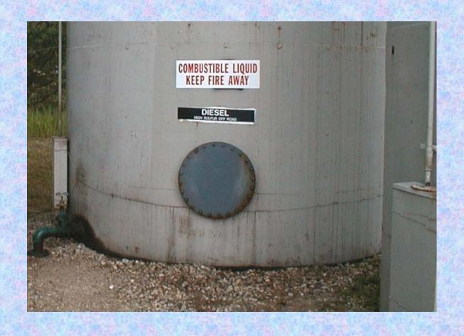
Single wall tanks resting directly on the ground are a concern!!
