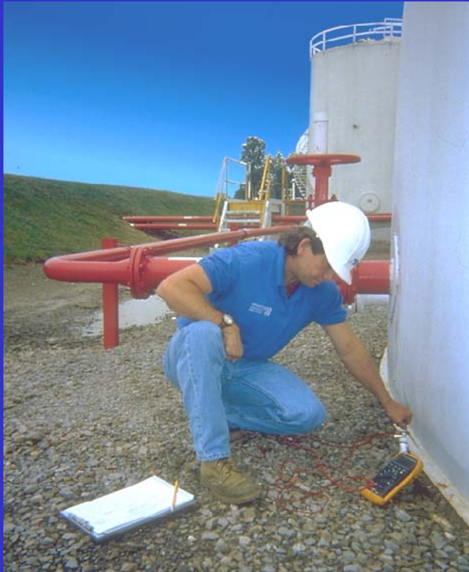
Annual Cathodic Protection Survey
