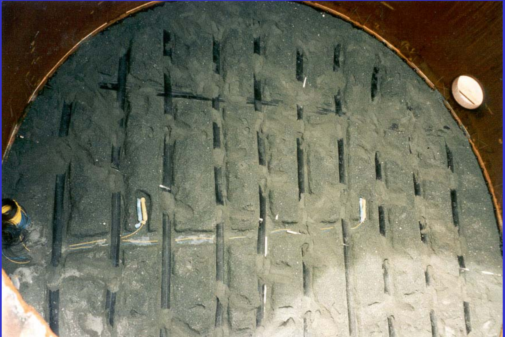
CP Installation on Rebottomed Tank
