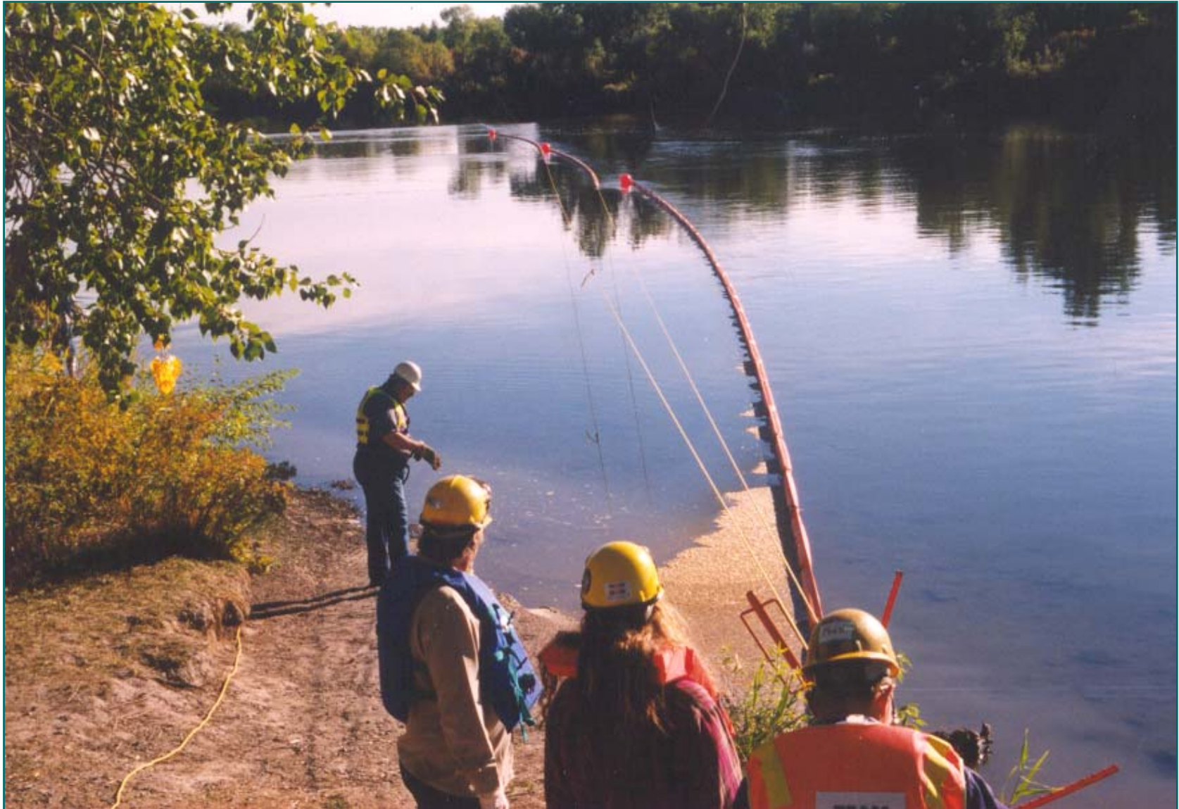
Bank to Bank Rope Anchor System Missouri River - Montana
