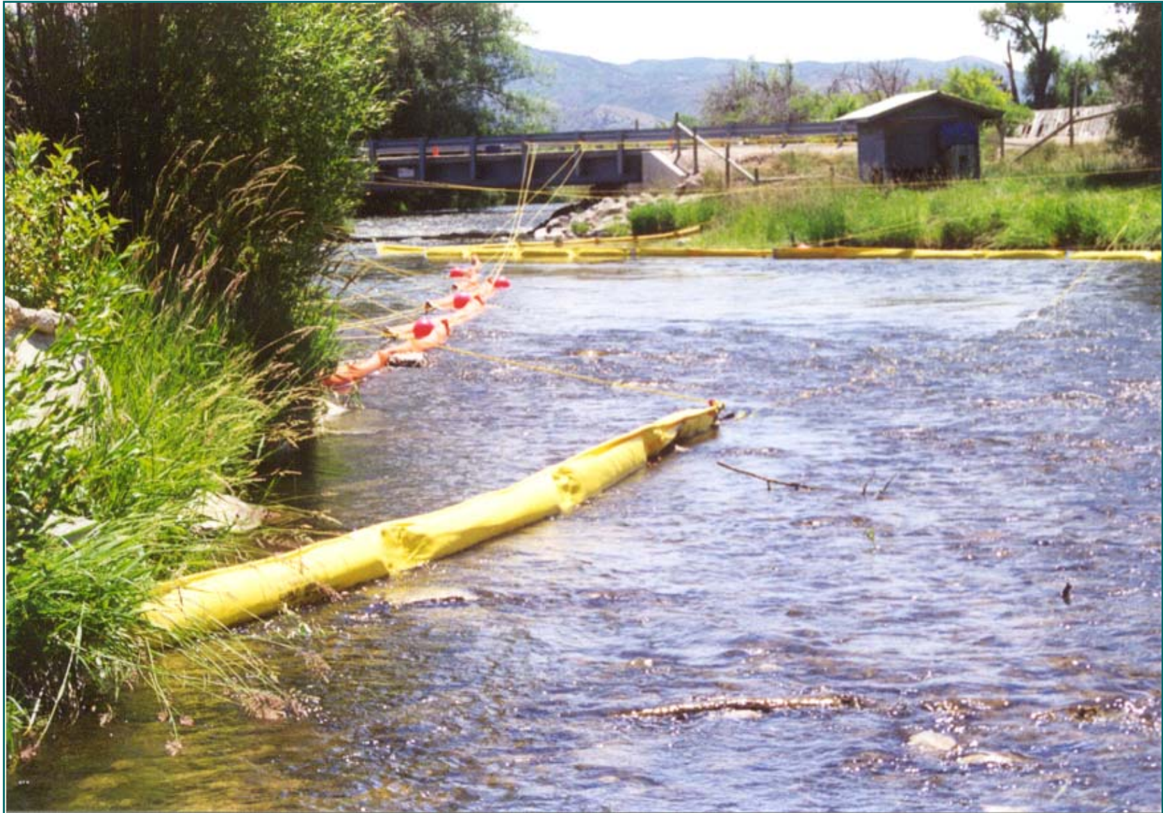
Bridge to Bank Rope Anchor System - View of Bridge Rope Anchoring Weber River - Utah
