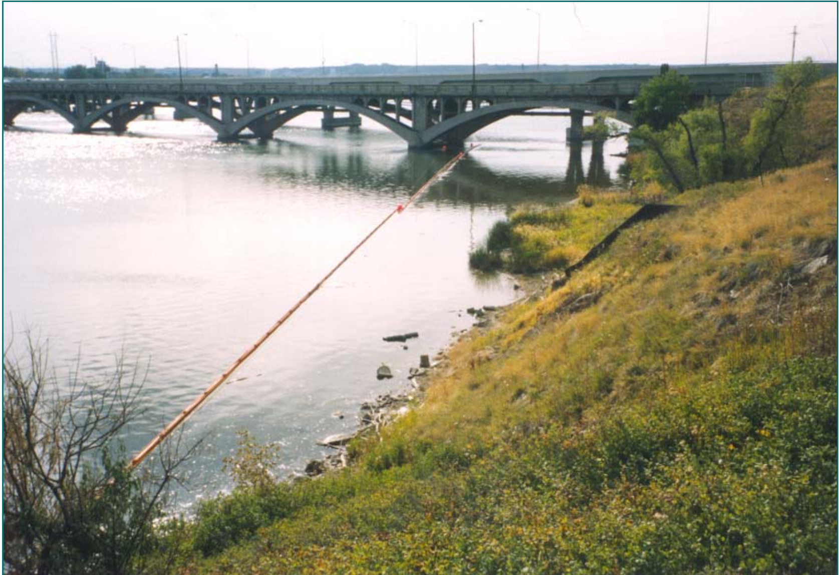
Bridge to Bank Rope Anchor System Missouri River - Montana
