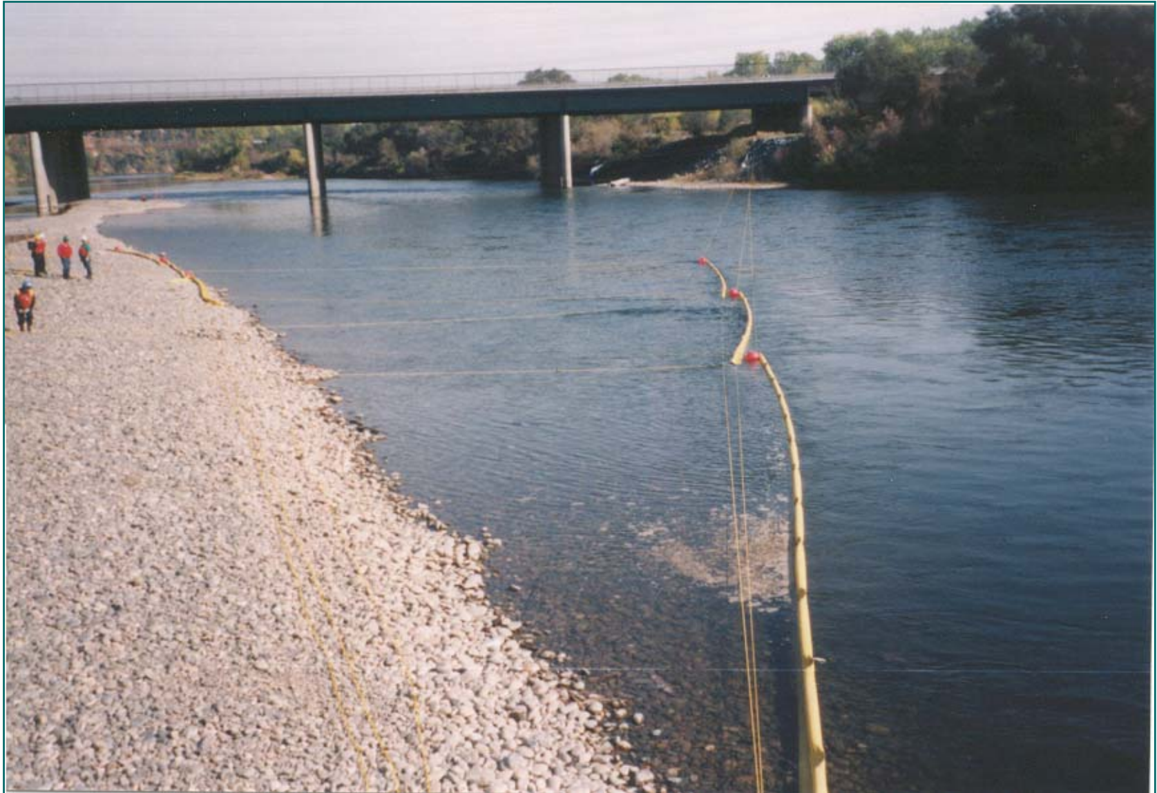
No. 3 - Boom Deployed - Bank to Bank Rope Anchor System American River - California
