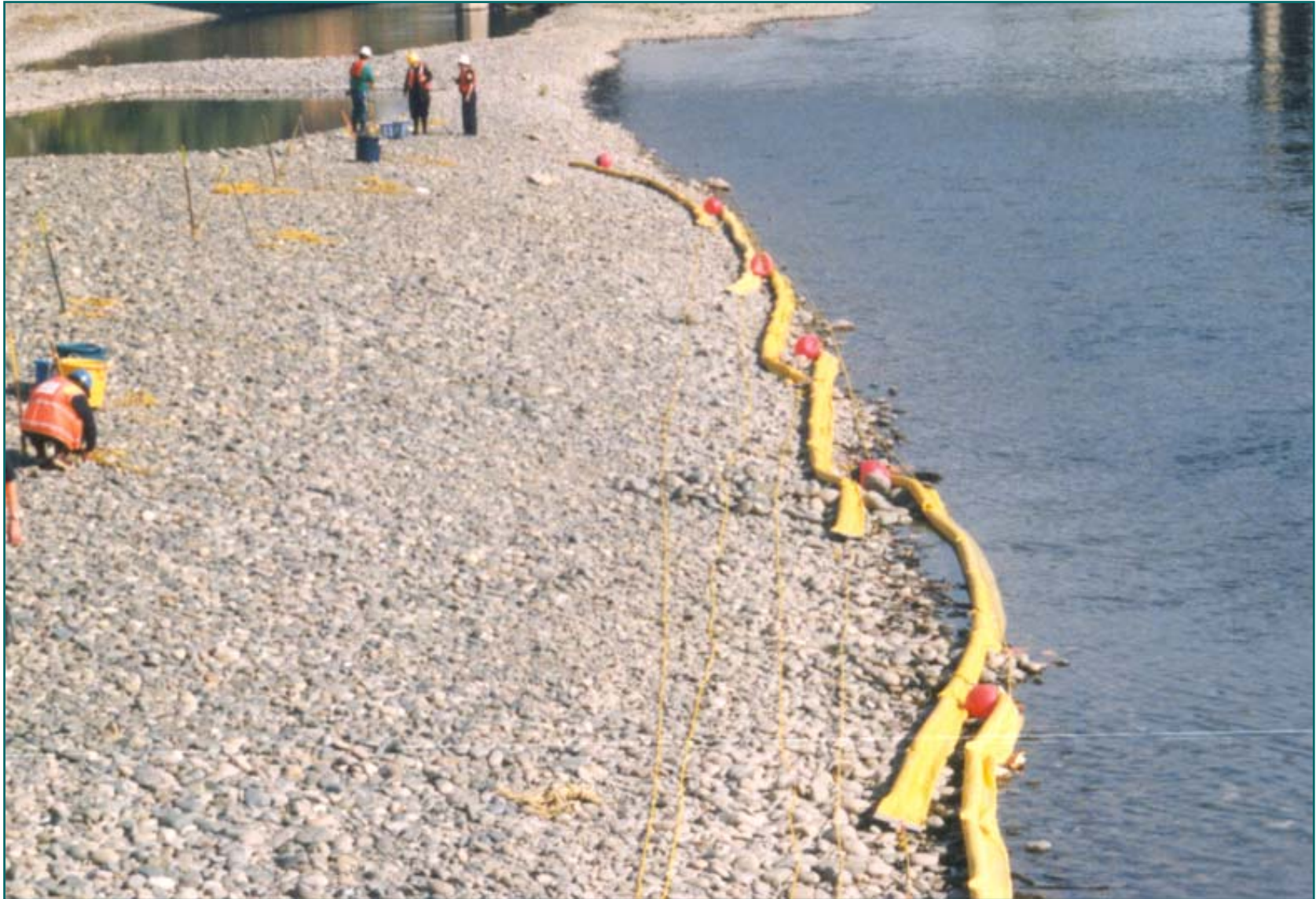
Bank to Bank Rope Anchor System - Bank Layout American River - California
