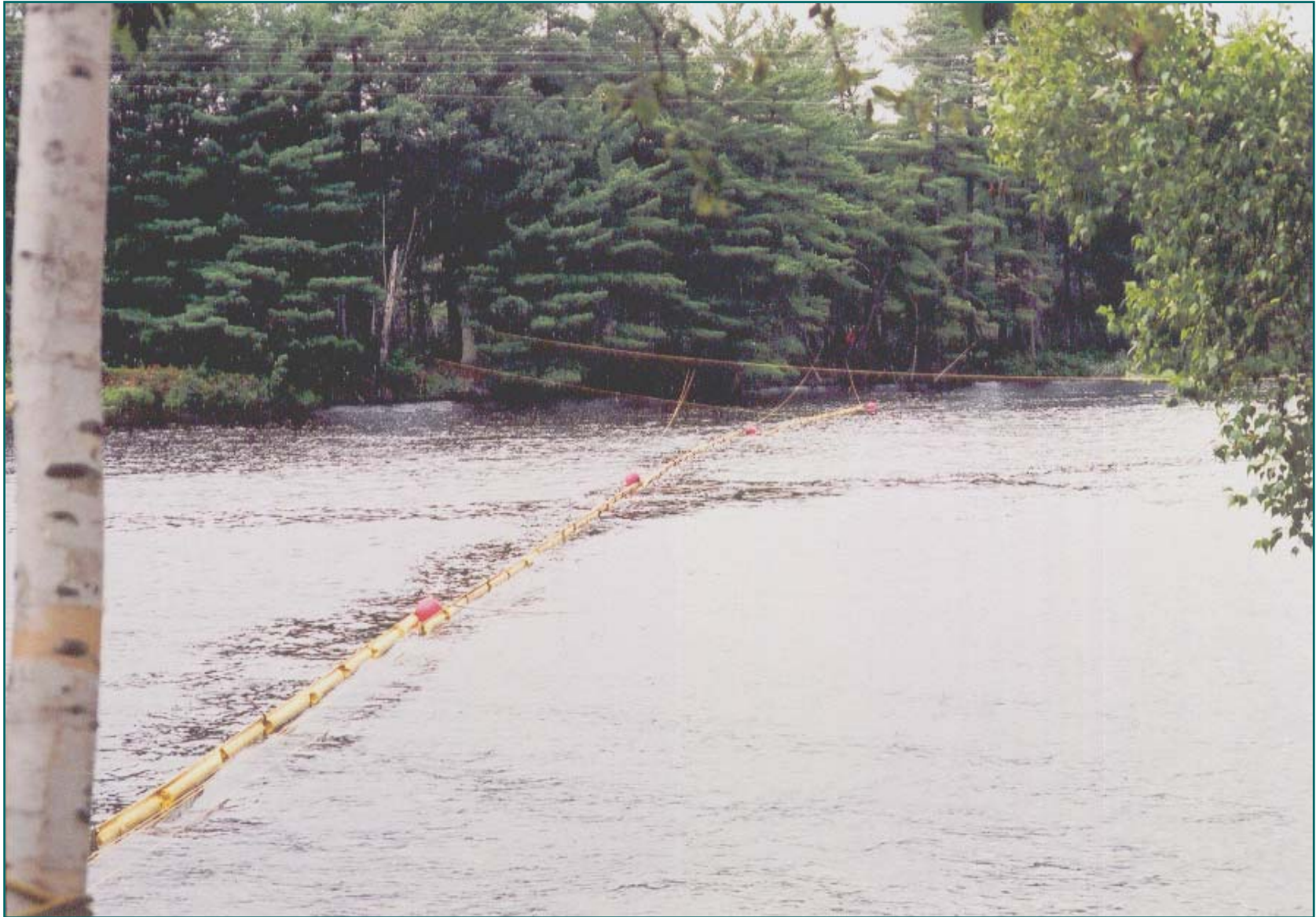
Bank to Bank Rope Anchor System Rio Grande River – New Mexico
