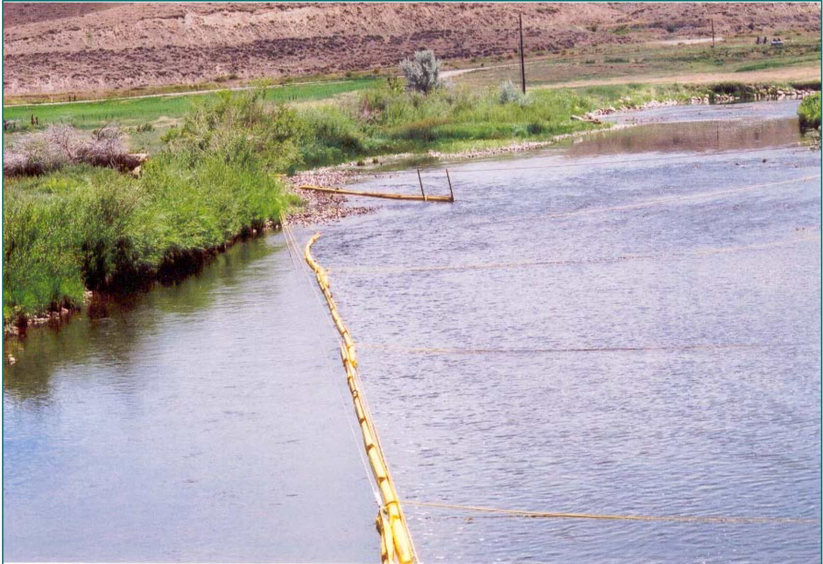
Deflection Booming - River Deployment Popo Agie River - Wyoming
