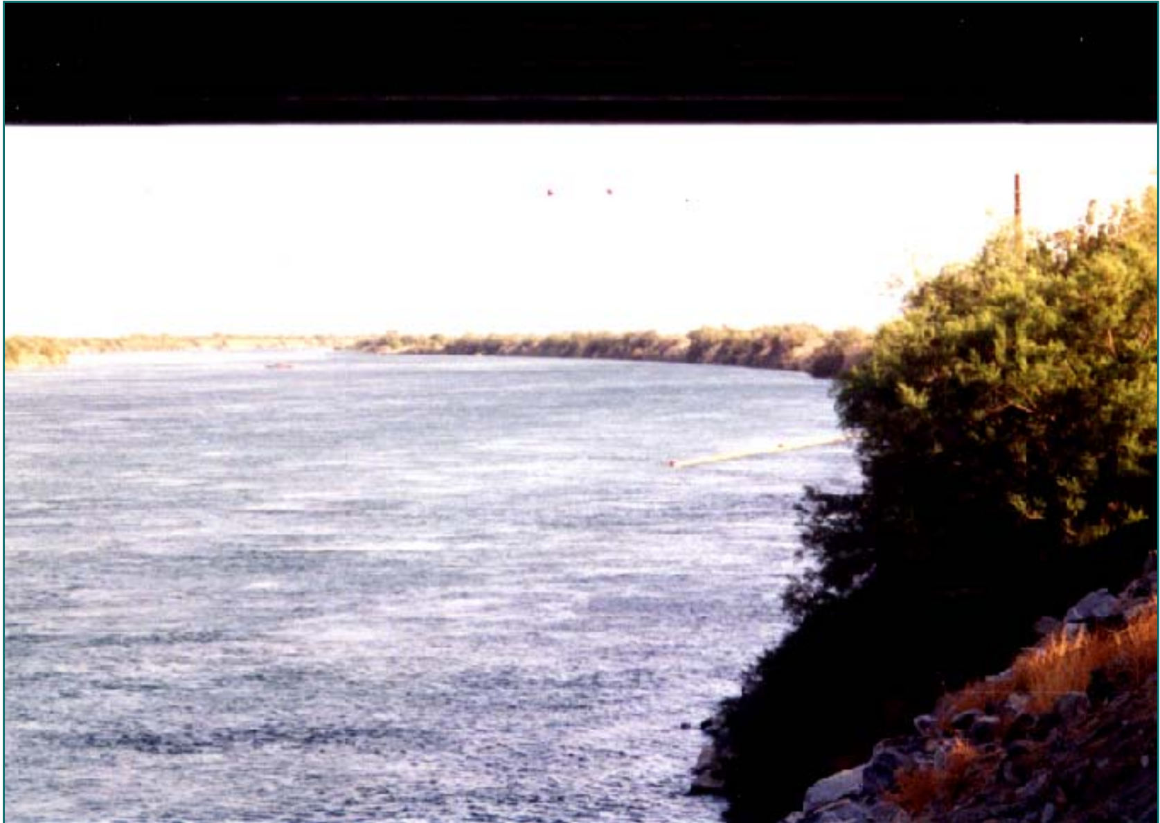
Bridge to Bank Rope Anchor System - View of Containment & Recovery Site Colorado River - Nevada
