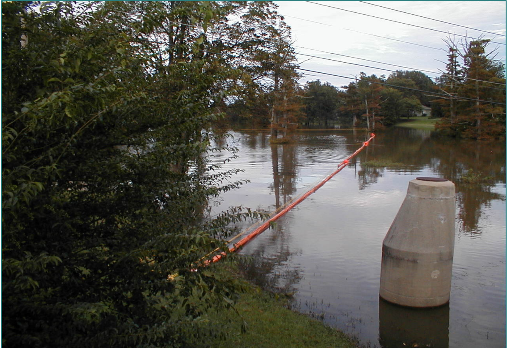
Cascade Diversionary Booming Modified Bridge to Bank Rope Anchor System (Trees)
