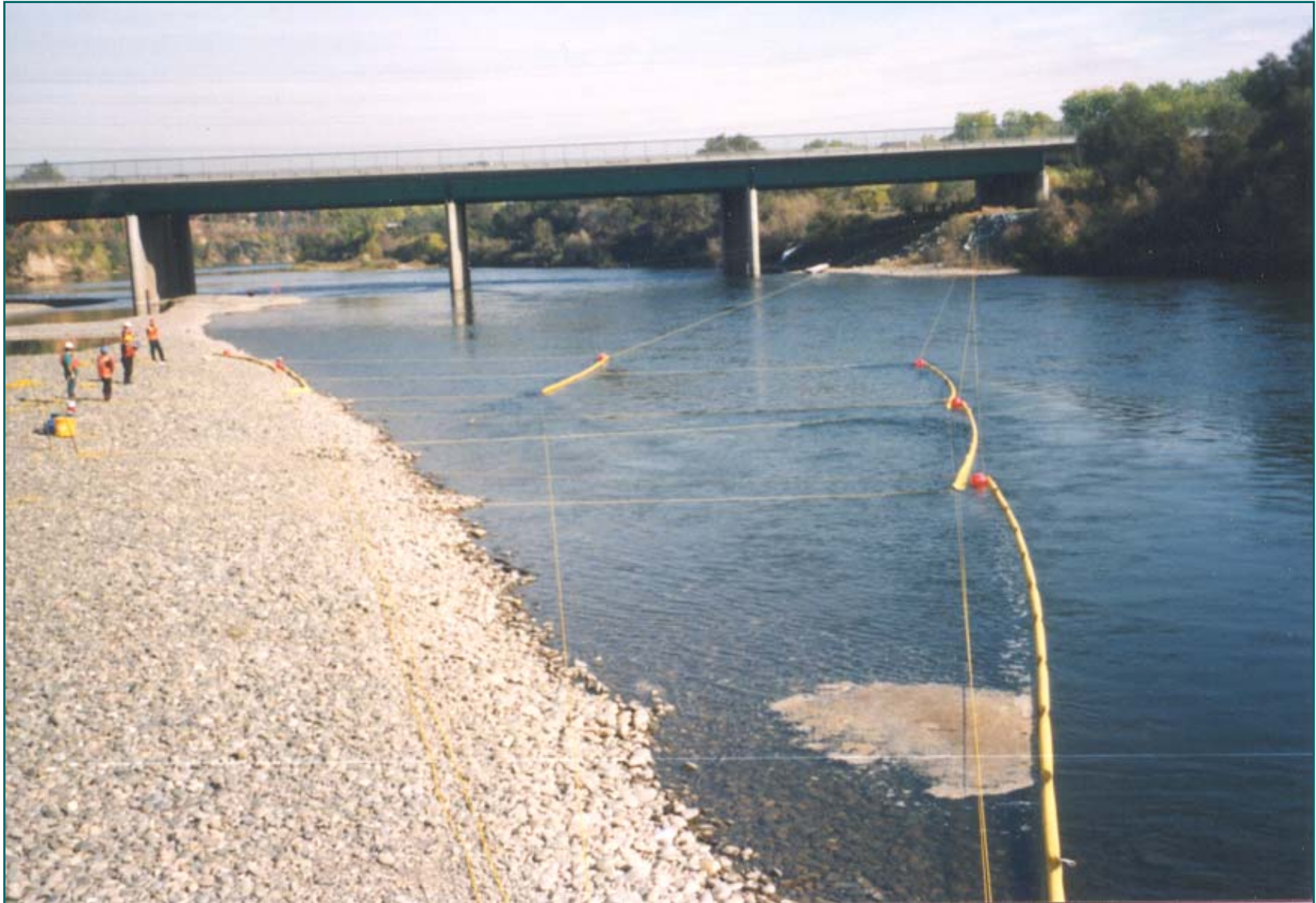
No. 4 - Boom Being Deployed - Bank to Bank Rope Anchor System American River - California
