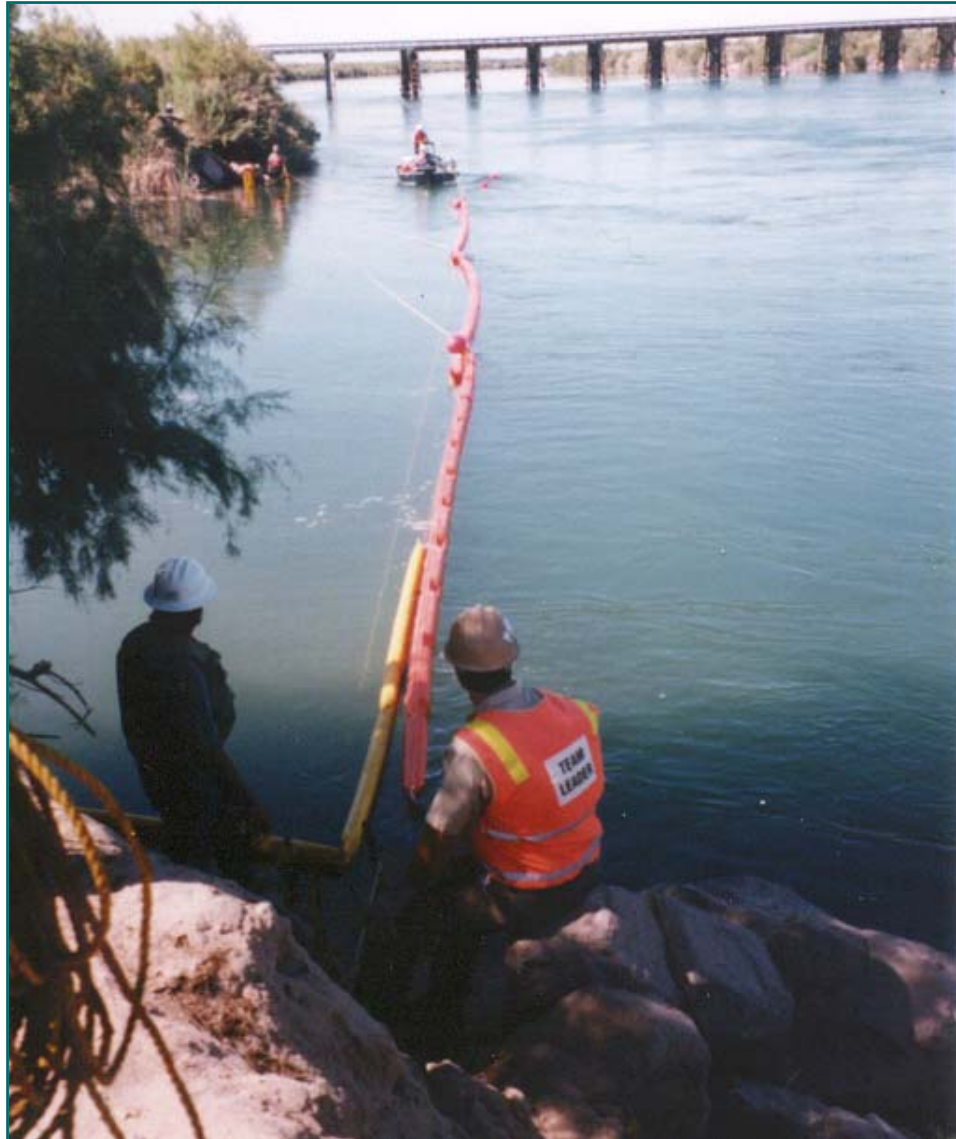
Bridge to Bank Rope Anchor System Boat deploying Rope Lead to Column "D" Ring & Shore Colorado River - California
