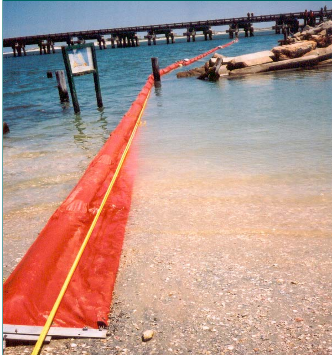
Bridge to Bank Rope Anchor System St. Johns River - Florida
