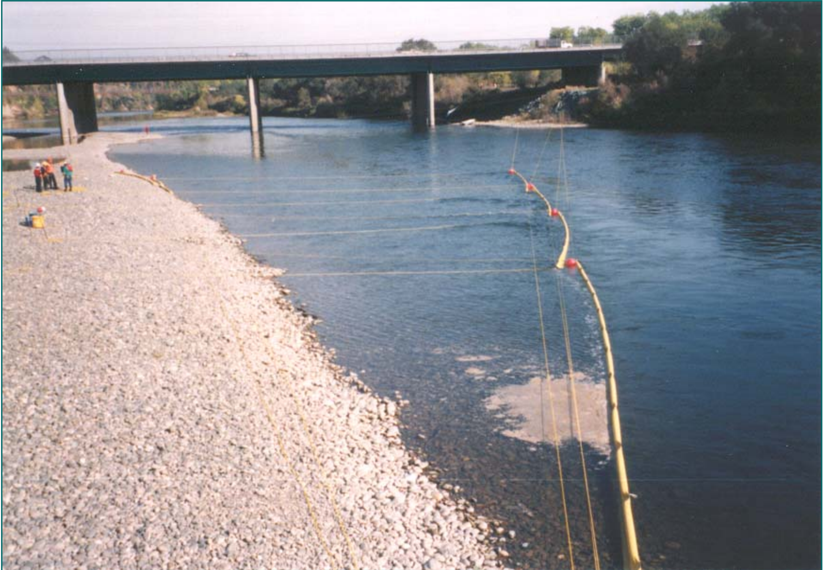
No. 4 - Boom Deployed - Bank to Bank Rope Anchor System American River - California
