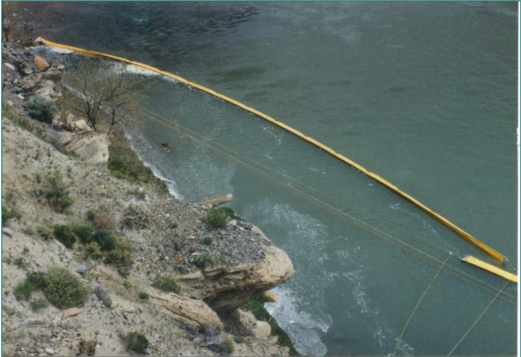
Containment Booming – Cascade System Shoshone River - Wyoming
