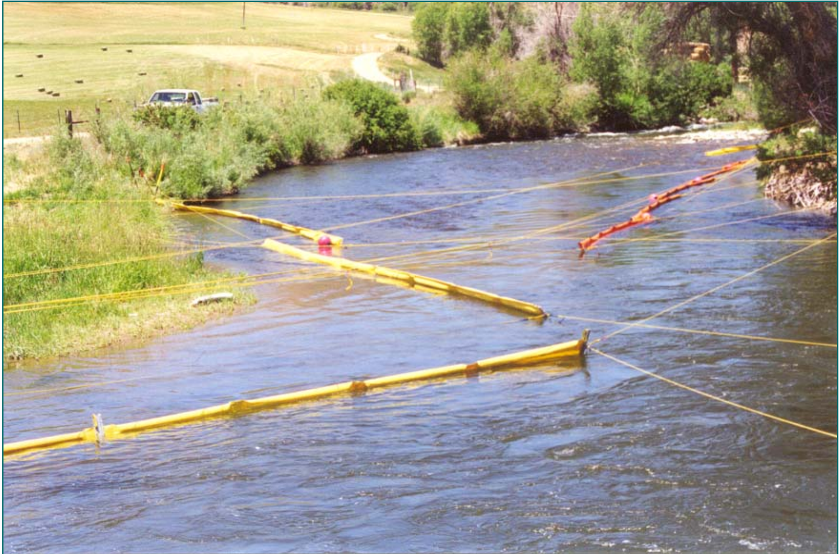
Bridge to Bank Rope Anchor System Open Chevron Cascade Boom Deployment with Deflection Weber River - Utah
