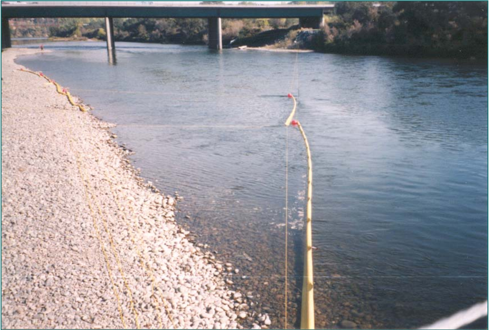
No. 2 - Boom Deployed - Bank to Bank Rope Anchor System American River - California
