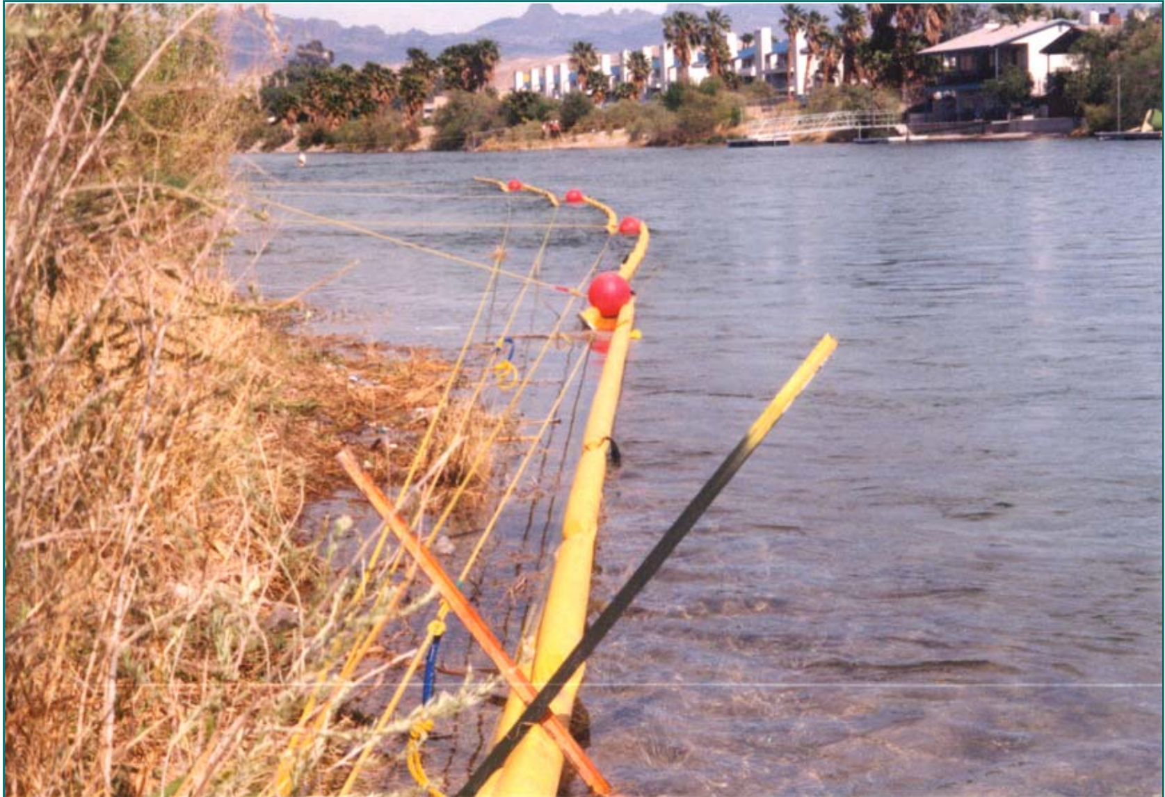
Bank to Bank Rope Anchor System Deployed Colorado River - Nevada
