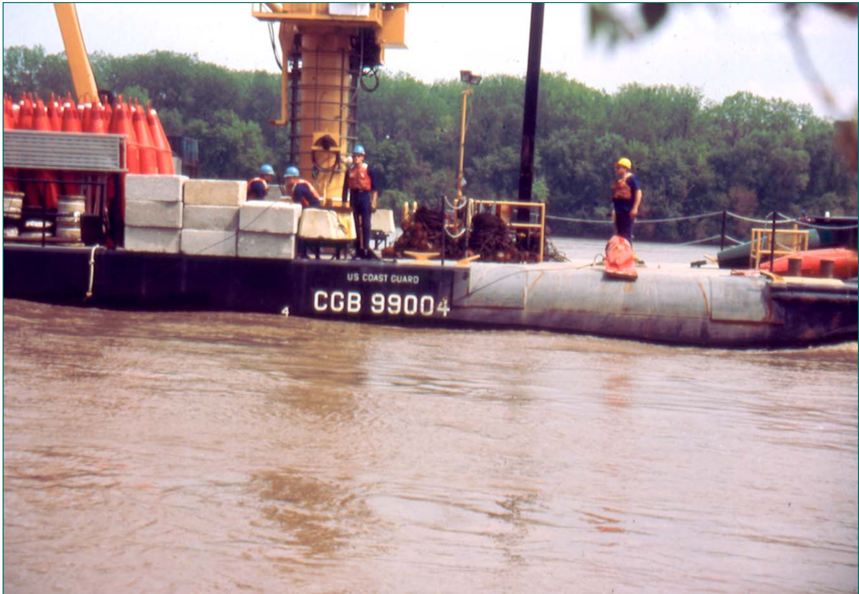
Buoy to Bank Anchor System USCG Buoy Tender in Position to Drop 1600 lbs. Sinker with Buoy Missouri River - Missouri
