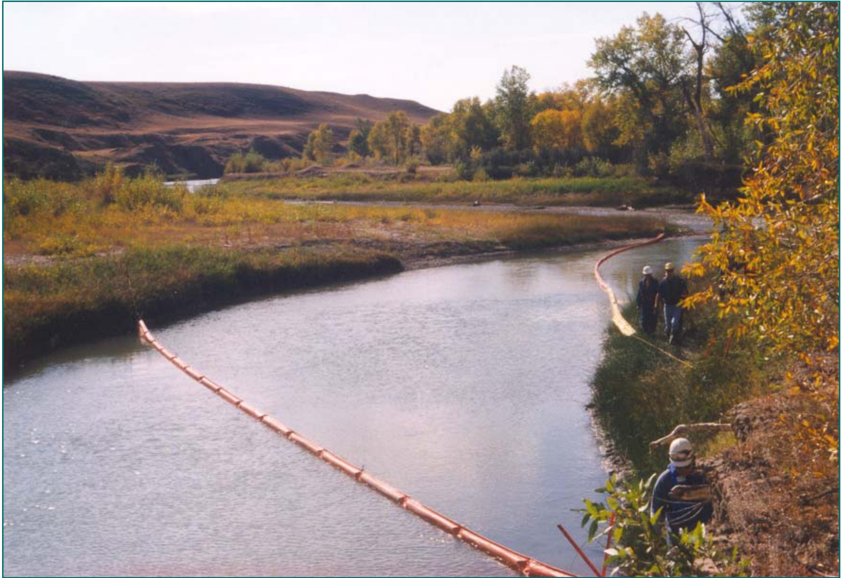
Single Diversionary Boom Deployment with Secondary Teton River - Montana
