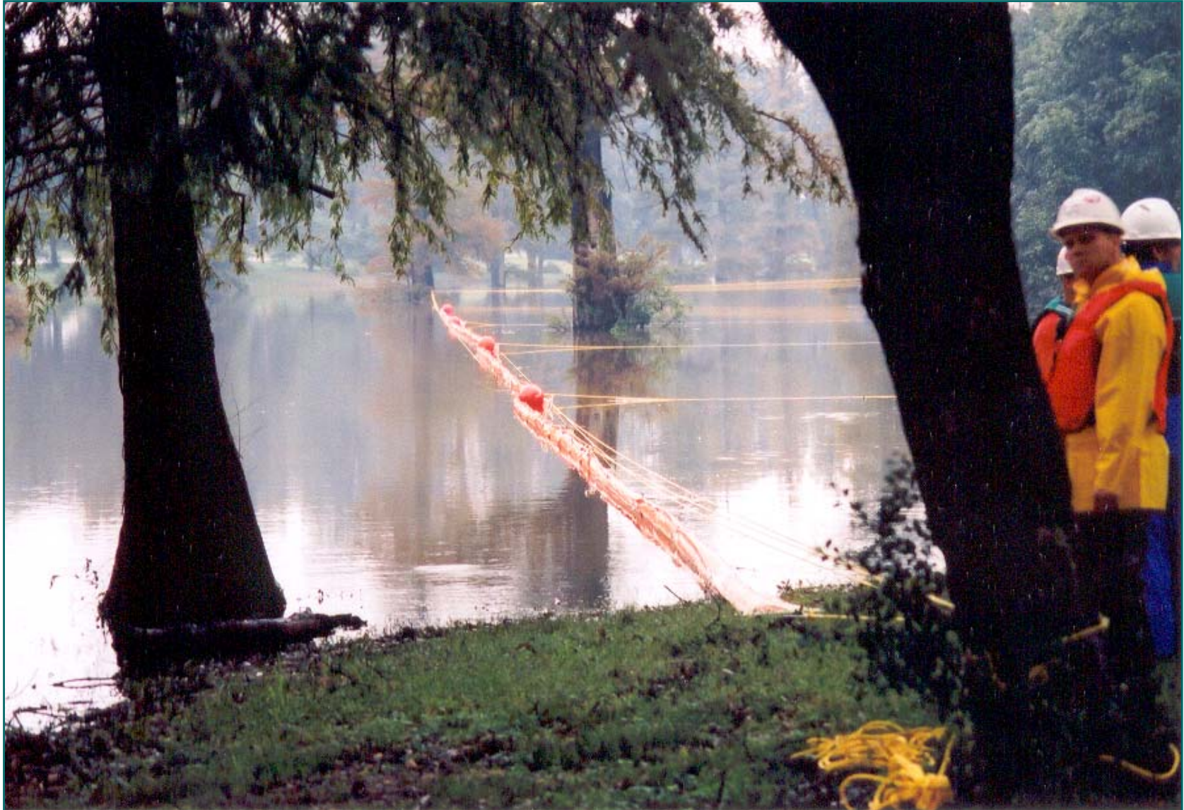
Modified Bridge to Bank Rope Anchor System (Trees) - Mississippi
