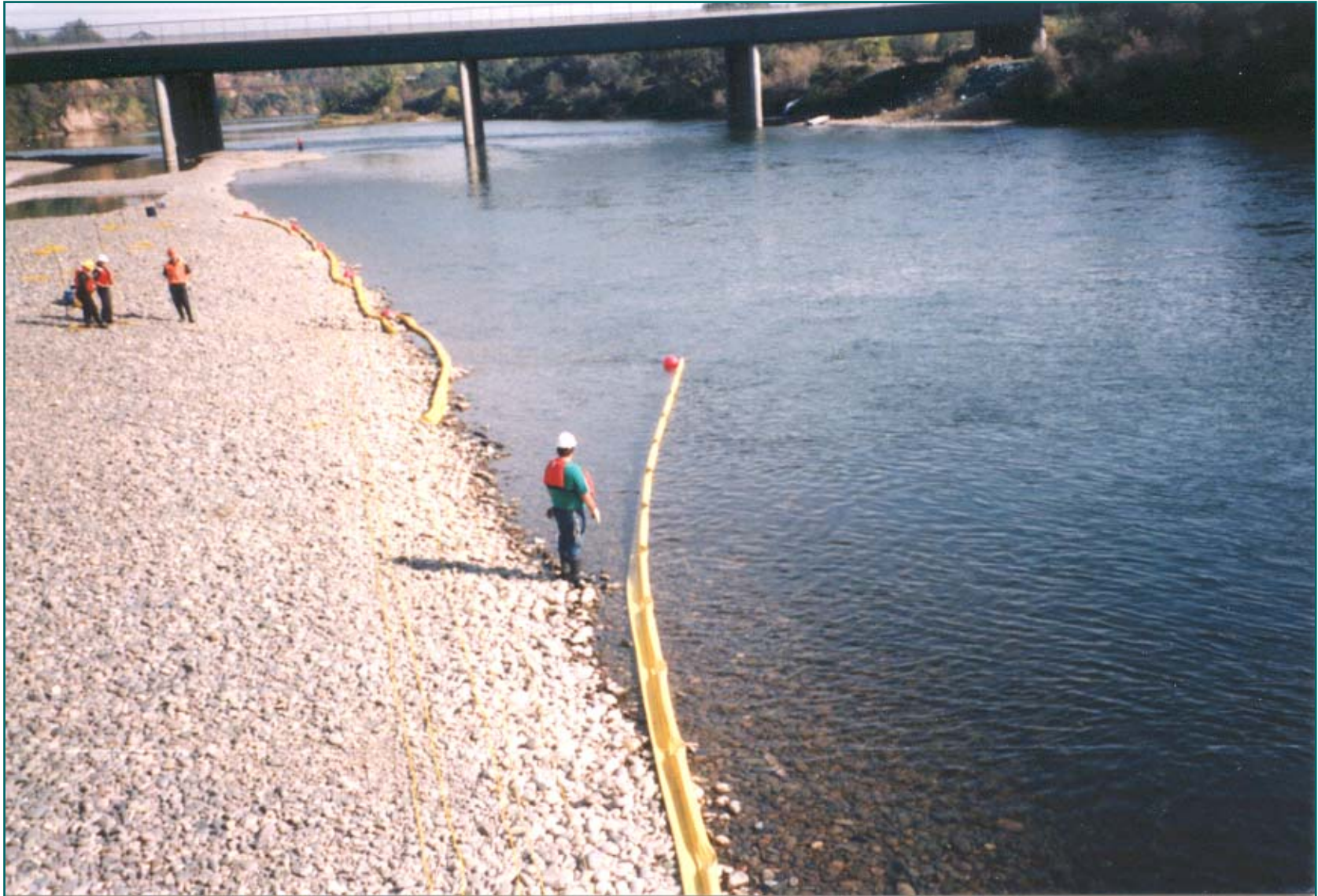
No. 1 - Boom Being Deployed - Bank to Bank Rope Anchor System American River - California
