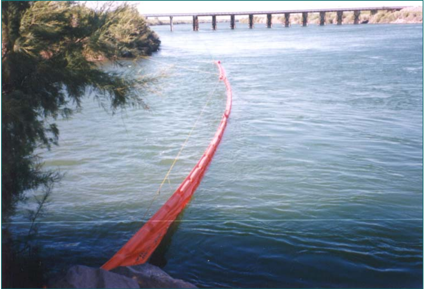
Bridge to Bank Rope Anchor System Colorado River - California
