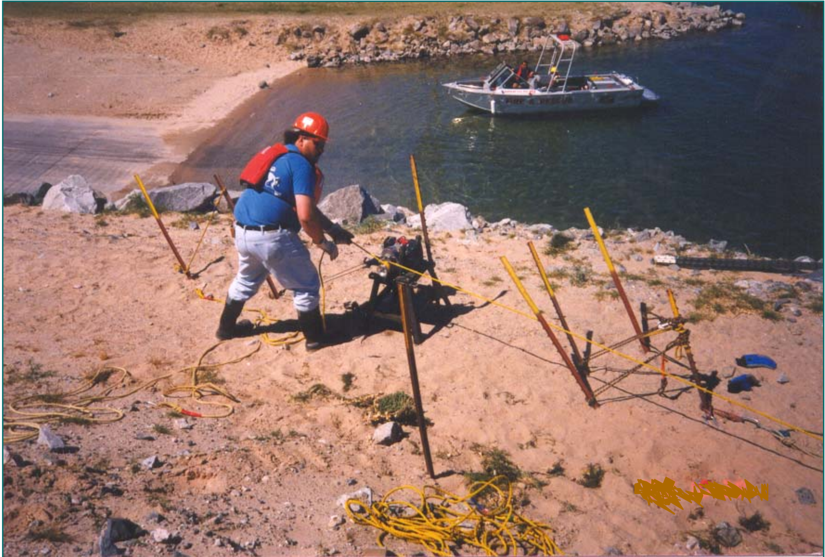
Rope Being Pulled by Power Winch with Side Capstan Mounted on Stand Colorado River - Nevada
