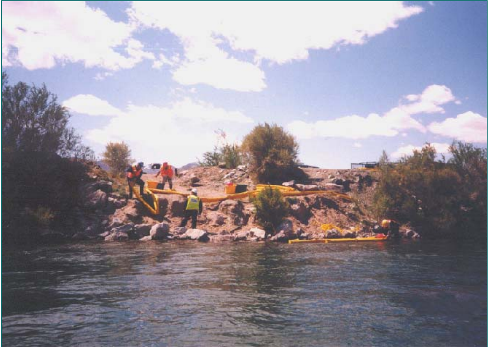
Bridge to Bank Rope Anchor System - Boom Layout on River Bank Colorado River - Nevada
