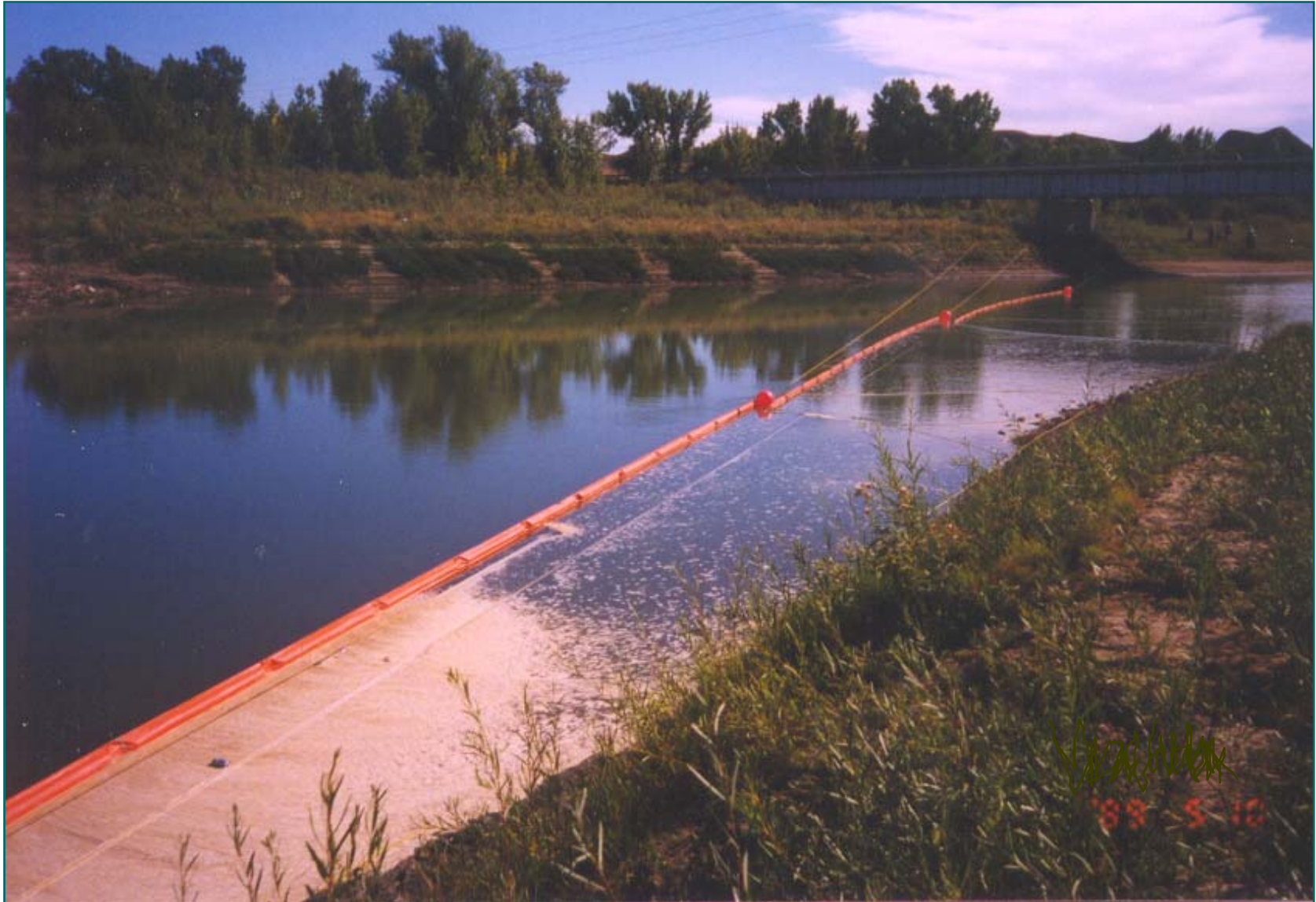
Containment Booming - River Bank Maris River - Montana
