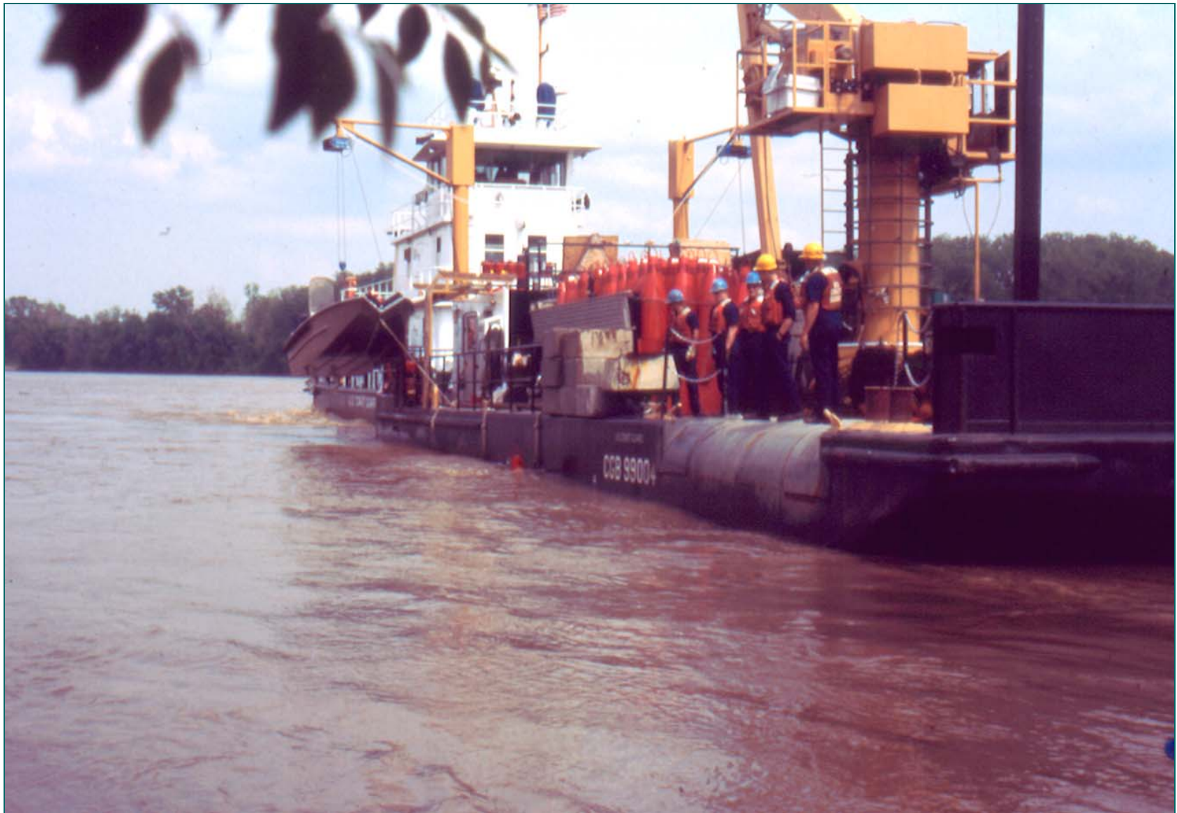
Buoy to Bank Rope Anchor System USCG Buoy Tender Dropping 1600 lbs. Sinker with Buoy Missouri River - Missouri
