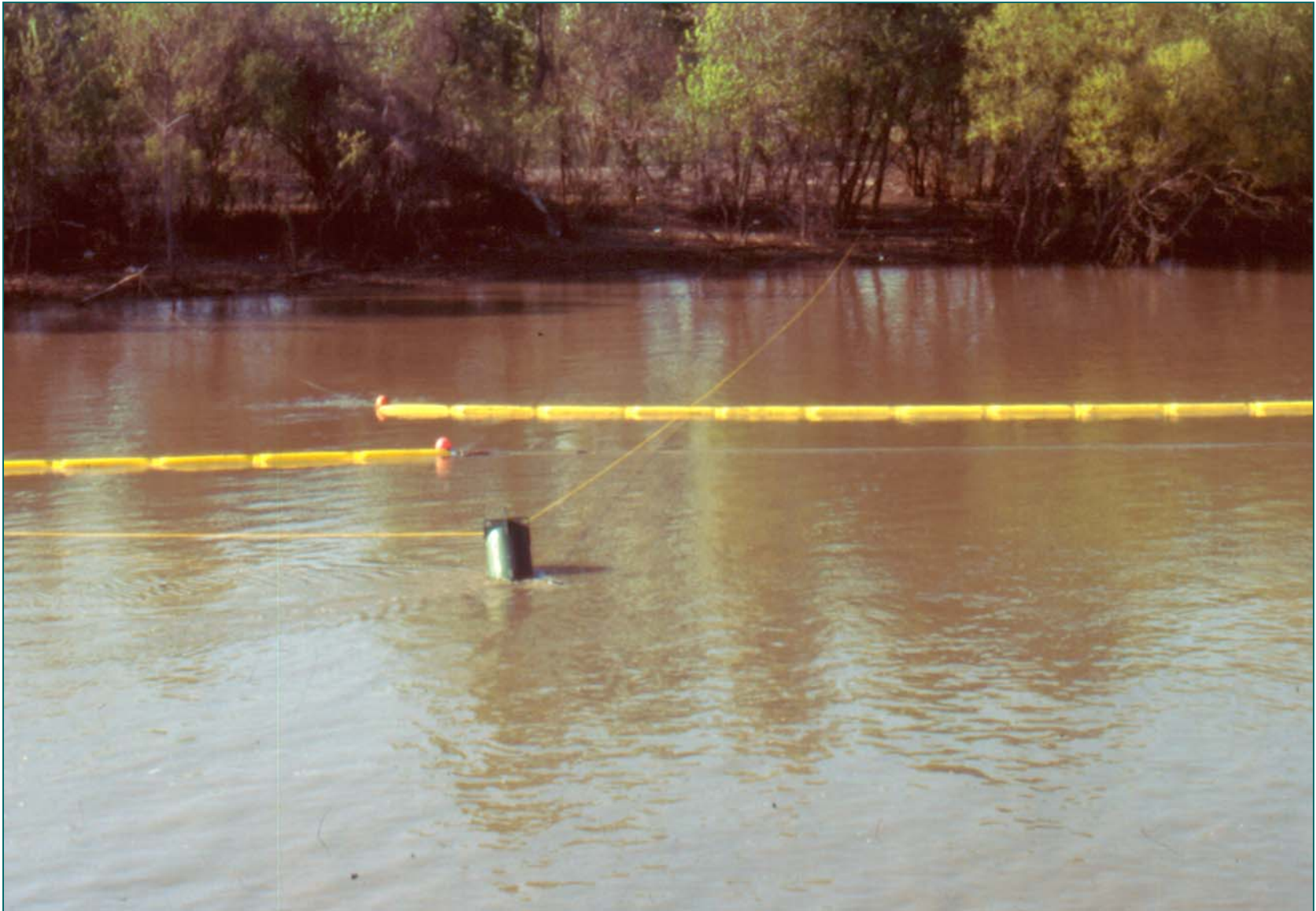
Buoy to Bank Rope Anchor System USCG Buoy Tender Dropping 1600 lbs. Sinker with Buoy Mississippi River - Missouri
