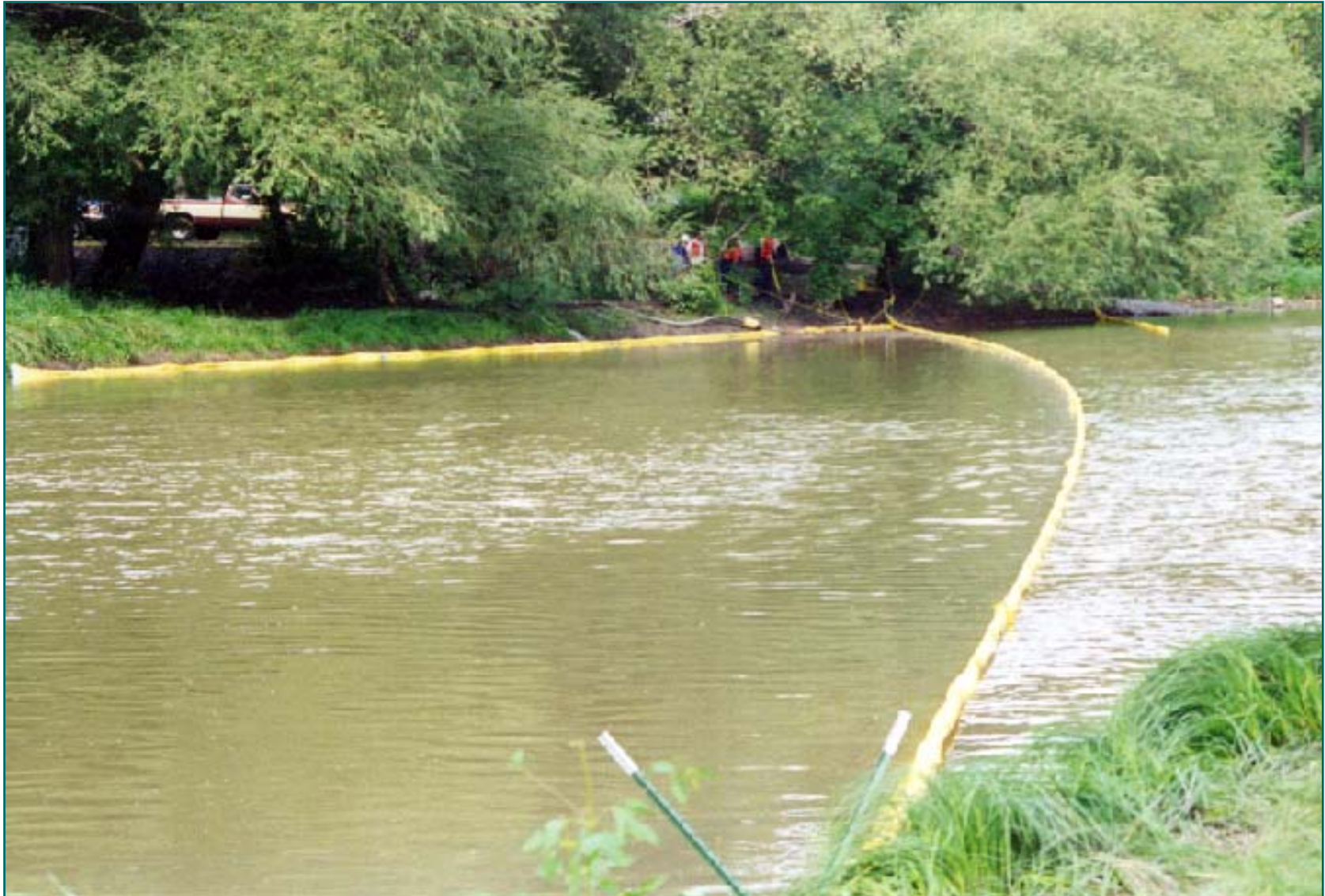
Single Diversionary Boom Deployment with Shoreline Protection Red River of the North
