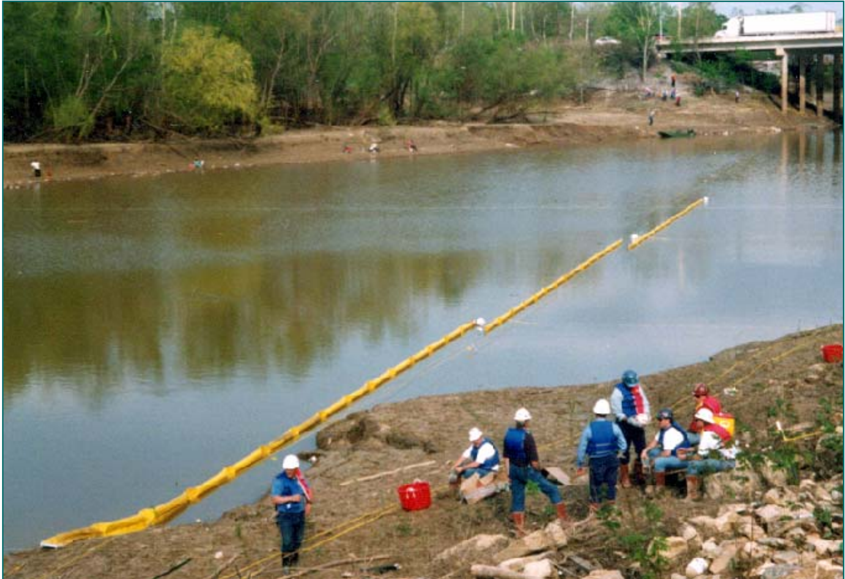
Bridge to Bank Rope Anchor System Nonconnah Creek - Tennessee
