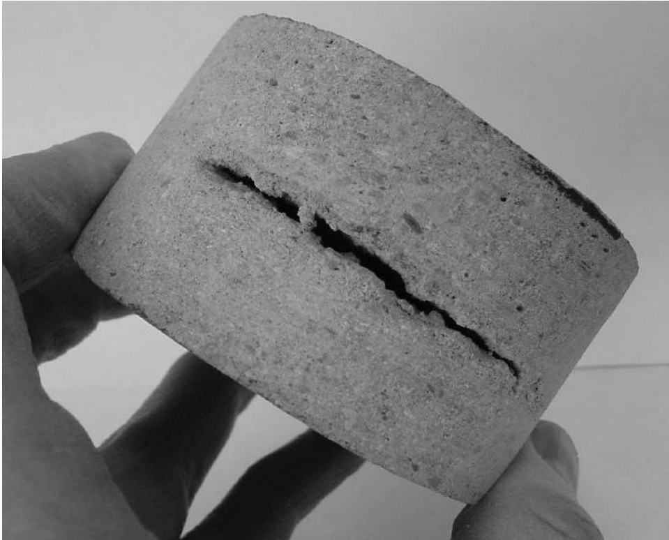
Figure 12 - Fine shotcrete coring with large void.
