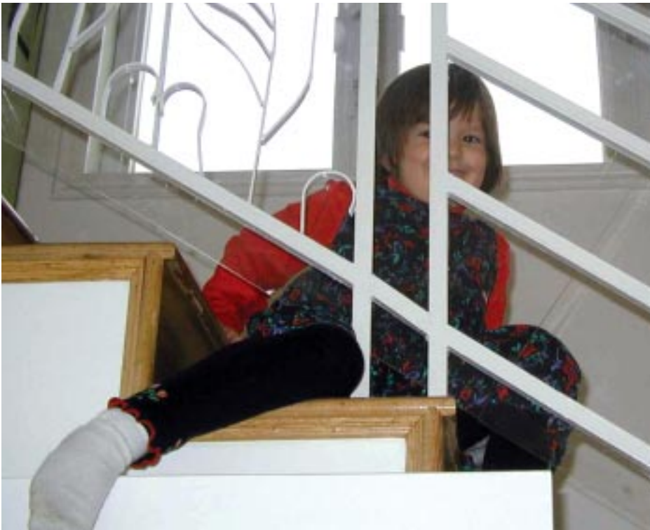
Above: A child demonstrates a guard installed over a risky railing at a Foreign Service officer's residence. Opposite page: Dennis Dubugras, a POSHO assistant at the U.S. Embassy in Brasília, Brazil, inspects propane tanks at a residence in Costa Rica as part of a training course.
