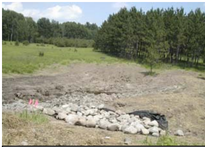
Figure 3. This is the Clark property immediately following construction in July 2005
