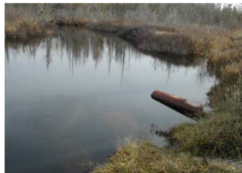
Figure 12. Robinson Road/Maple River crossing before construction.
