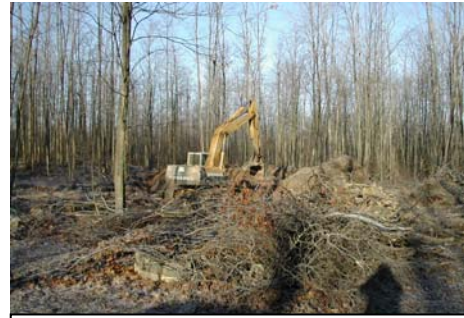
Figure 7. Westenbarger property, during construction December 2004
