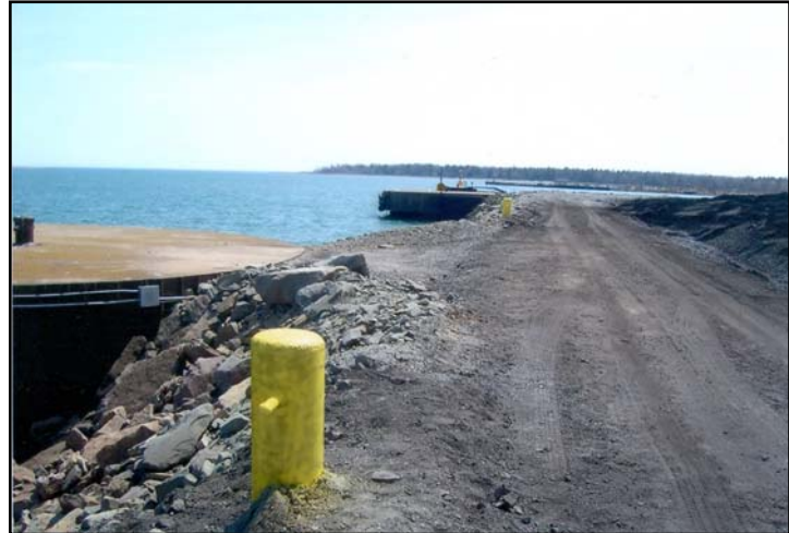
New tie off pilings (foreground) installed at Detroit Edison (DTE) Harbor Beach Power plant by Rooney Contracting to aid in securing stocking vessel M/V Spencer F. Baird. Photo credit: Ken Merckel.
