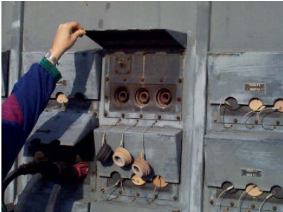
Figure 13-5. Skid-Mounted Substation with Single-Pole Connections
