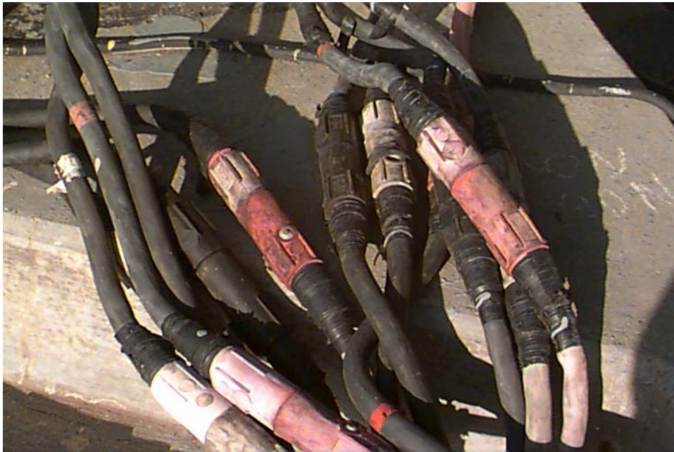
Figure 13-11. 480 Volt Shore-Cable to Ship-Cable Plug and Receptacle Connection In Place
