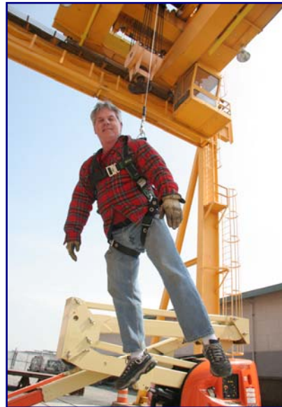
NSA rigger Paul Kerr tests out self-retractable lifeline fall protection recently installed to protect riggers on a 200-ton overhead bridge crane.
