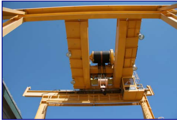
200-ton Ederer overhead bridge crane at the Naval Support Activity Mechanicsburg before it was outfitted with self-retractable lifeline fall protection devices.
