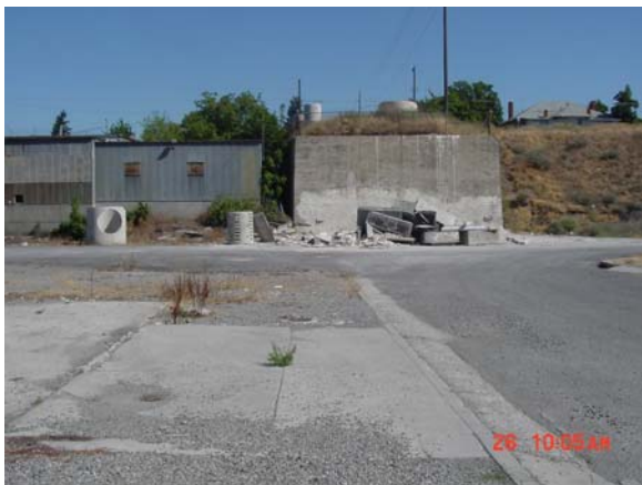
View of bluff and cement bridge abutment. Roof of residential home can be seen in top right. July 2001
