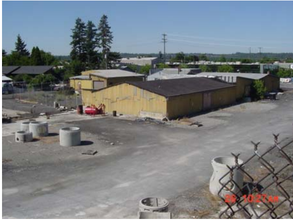
Warehouse buildings as viewed from top of bluff. July 2001
