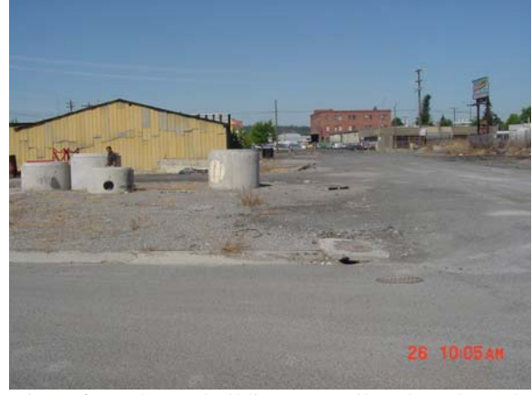
View of warehouse building near railroad grade. July 2001.
