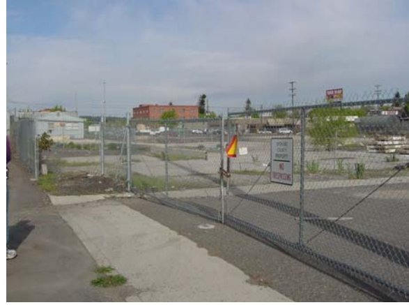
View of site after buildings were demolished. The only structure remaining is the gray structure on the center left. May 2003.
