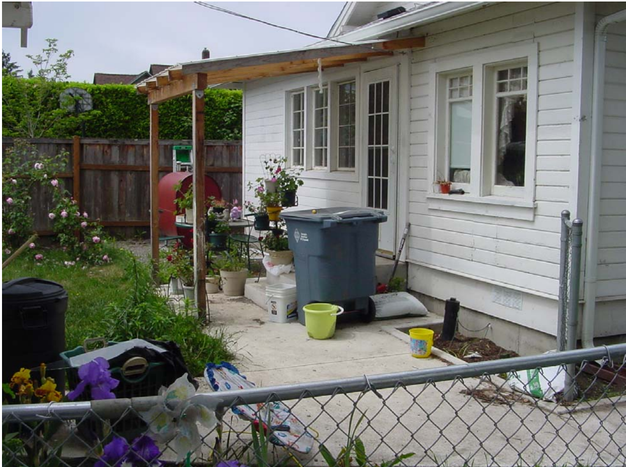
Figure 3. Patio view of site, after remediation.
