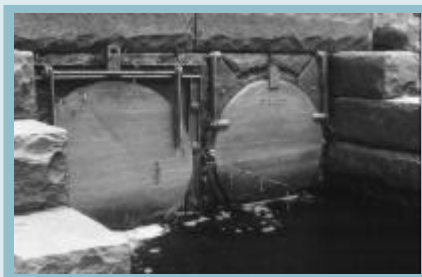
Tidegates deprive salt marshes of essential tidal flow. These gates, on Back River Creek, Woolwich, ME have been removed.
