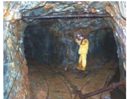
An inspector checks on conditions at junction of two tunnels deep within Holden Mine.
