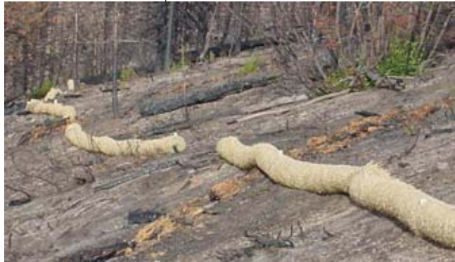
Terracing with straw 'wattle' bundles to minimize mudslides and erosion in the Safety Harbor Creek area
