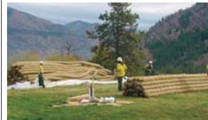
Straw 'wattle' bundles stacked up and ready for transport to the burned area.
