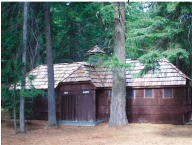
American River Lodge gets a new roof
