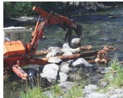
Fish habitat improvement involving placement of large wood in the Entiat River. Photo by Joe Kelly, USDI BLM
