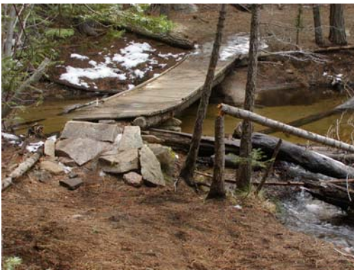
Before: Beaver Creek Trail Bridge with inadequate soil erosion measures and failing structure.
