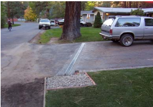
Slotted drain and drywell to infiltrate driveway runoff on a residential property.
