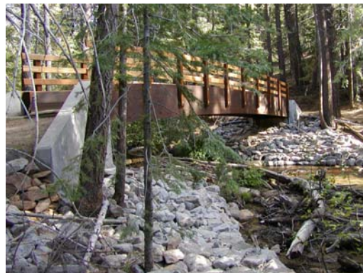
After: Beaver Creek Trail Bridge with larger flow area, improved soil erosion measures, and safe structure.
